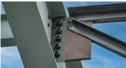
Flush-frame connection designed for efficiency
