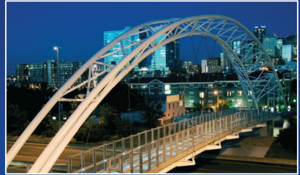
2007 NSBA Special Purpose Prize Bridge Award - 152 tons of 18" pipe curved in our Kansas City plant for the Highland Bridge. Denver, CO
