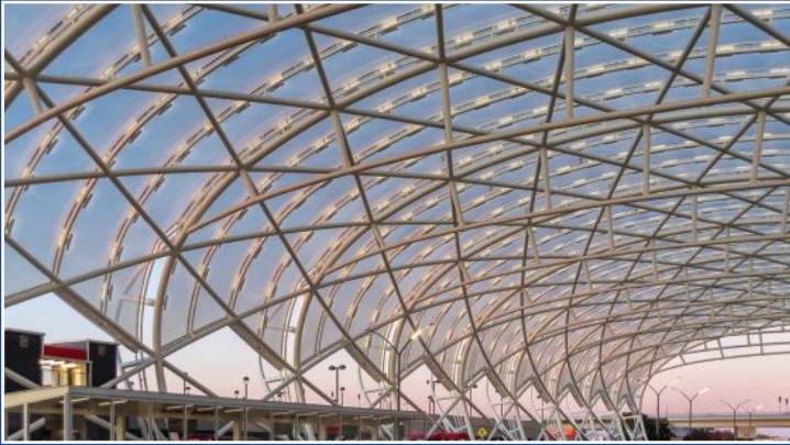
2020 IDEAS 2 National Winner - 920 pipe members rolled from 1300 tons of 14" pipe creating 38 super-trusses for the iconic canopy at Hartsfield-Jackson Atlanta Intl Airport. Atlanta, GA
