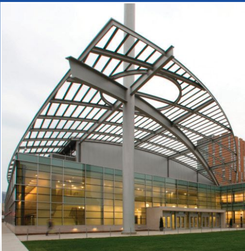
2010 NCSEA Award Winner - 200 tons of beams, channels and angle for the roof of the University of Illinois at Chicago Forum. Chicago, IL
