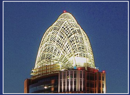
2012 IDEAS 2 Merit Award - 133 tons of 16" pipe curved for the Rooftop Tiara of the Great American Tower at Queen City Square. Cincinnati, OH
