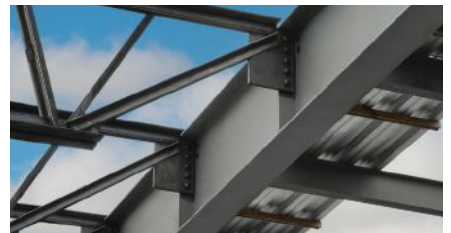
Joist reaction point occurs at beam centerline
