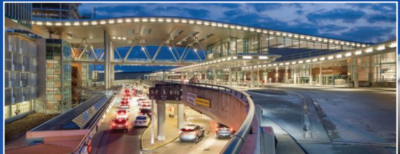
2024 IDEAS 2 Excellence in Engineering Award - Curved W36x182 beams the hardway against their strong axis and W36x135 members in a complex compound reverse s-curve (multi-radial) easyway against the weak axis at the Nashville International Airport. Nashville, TN
