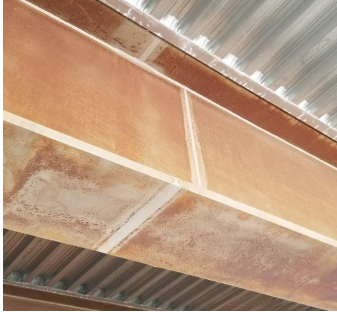
Figure 19. Steel plate girder with flange-to-web welds intersecting CJP groove welds in butt joints used to accomplish flange and web shop splices.
