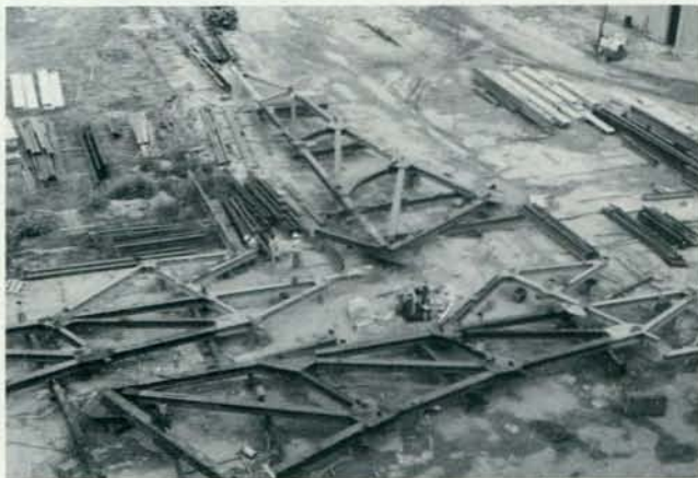
The large trusses were assembled on the ground to very tight tolerances. Safety nets were attached to the trusses with twin cables and pulled into position before the iron workers were allowed onto the trusses, which were erected 100' in the air.
