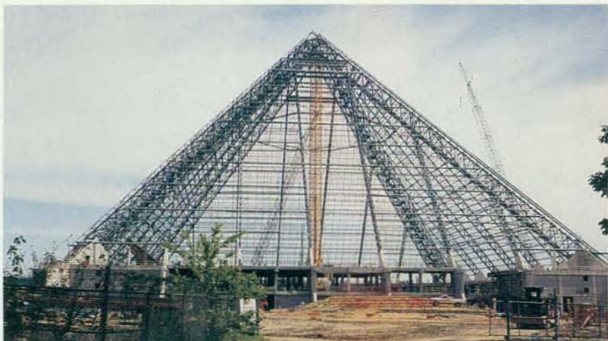
The Pyramid Arena in Memphis is a unique steel framed structure. Joists were used as part of the support system for the skin of the building.
