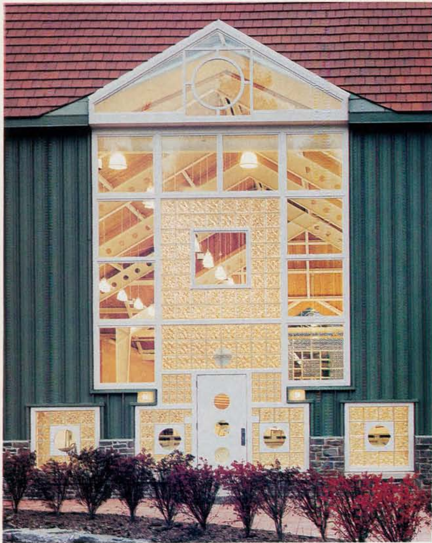
A view from inside and out: Letting in a huge amount of natural light was crucial to the designer's plan for the Hamilton College Pool. Just as important was the use of steel three-hinged arches for the structural system, which allowed both the required 53' head room and 65' clear span. Photography by Richard Mandelkorn © 1989
