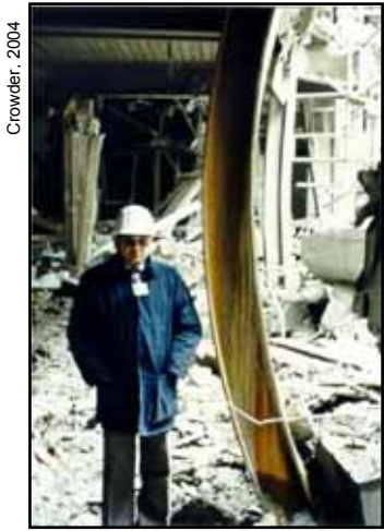
Figure 1.11 Ductile Column Response to Blast
