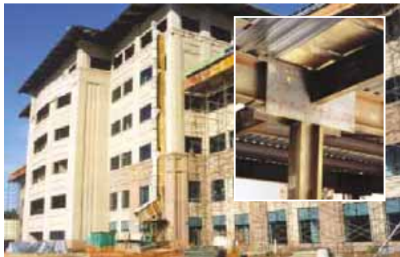
Figure 3.1 Pacific Command Center and Proprietary Blast-Resistant Connection Detail
