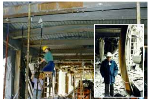
Figure 7.7 Exchequer Court, St. Mary’s Axe, City of London
