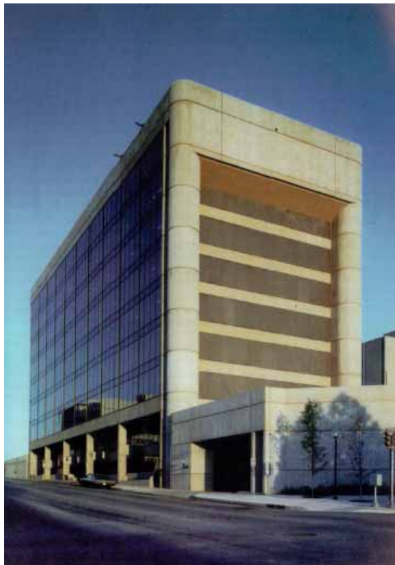
Figure 1.2 Oklahoma City Federal Building Prior to Attack
