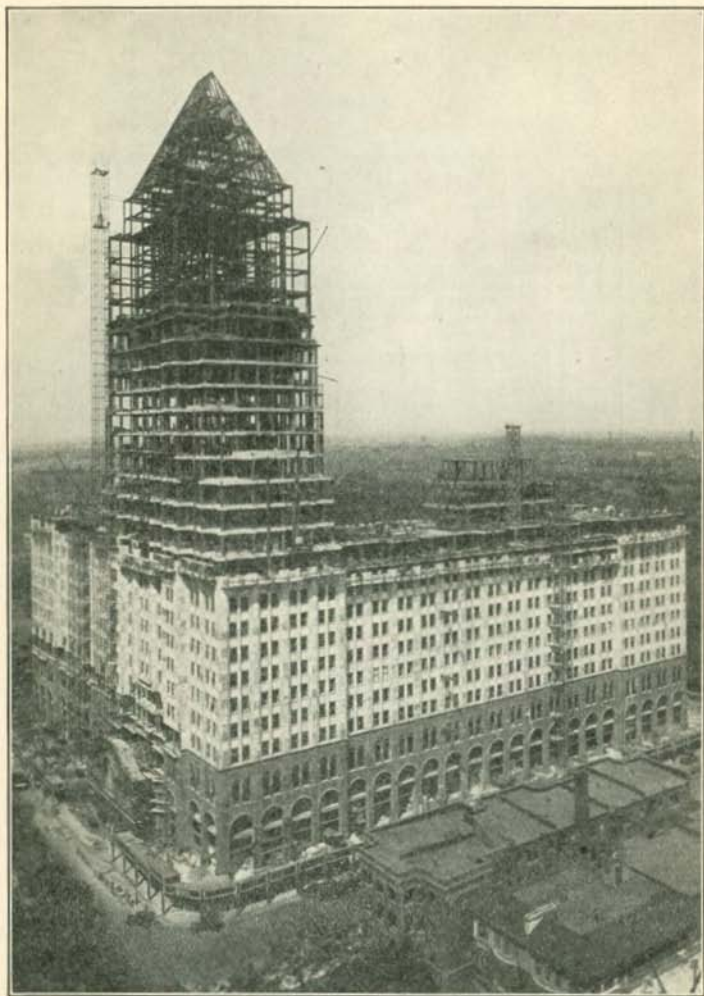
FISHER BUILDING—DETROIT, MICH. CARNEGIE BEAM SECTIONS IN STEEL CONSTRUCTION
