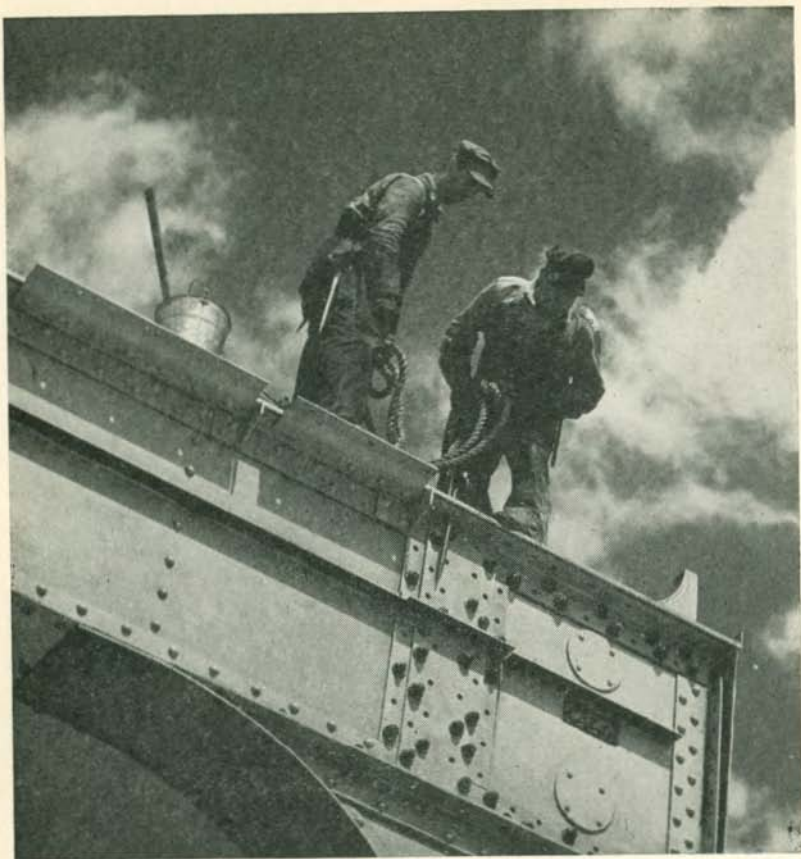
Inland Structural Steel at Work
