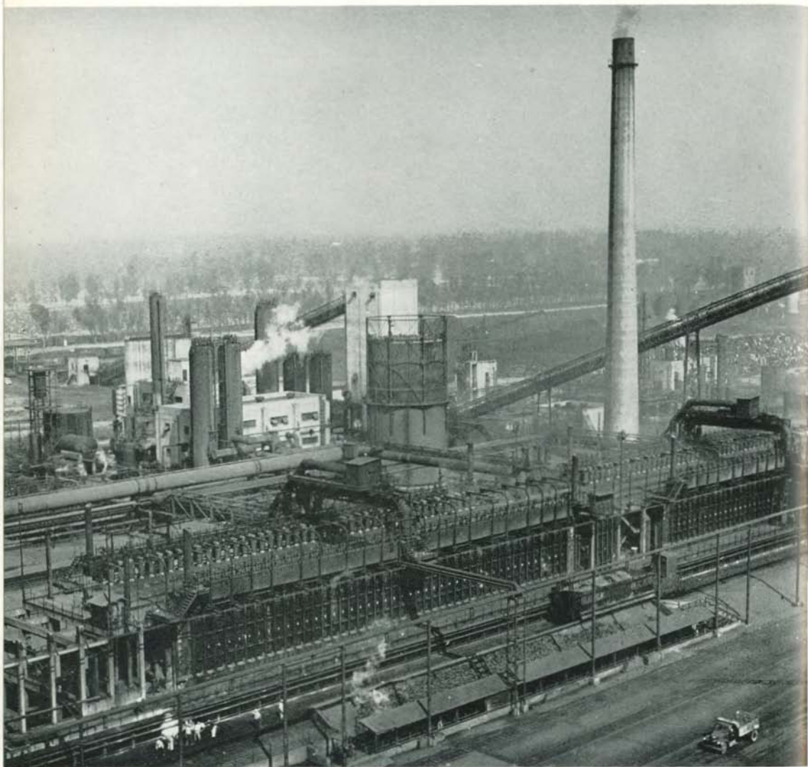
Volatile-bearing gases from the coke ovens are processed in by-products plant (background) for the recovery of creosote oil, ammonium sulphate, phenol, benzol and other chemicals.
