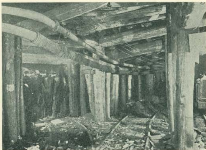
Heavy Wooden Timbering, Anthracite Mine
