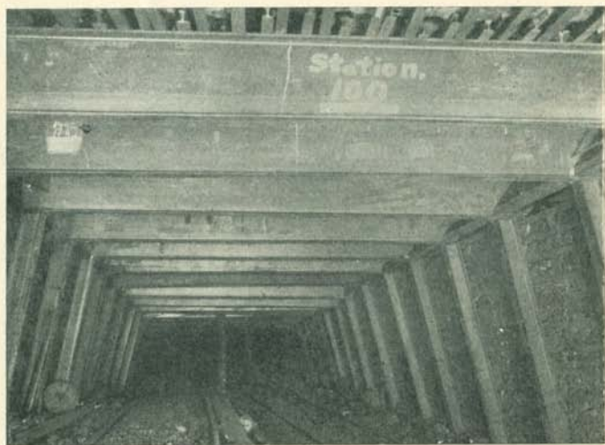
Heavy Steel Timbering, Anthracite Mine
