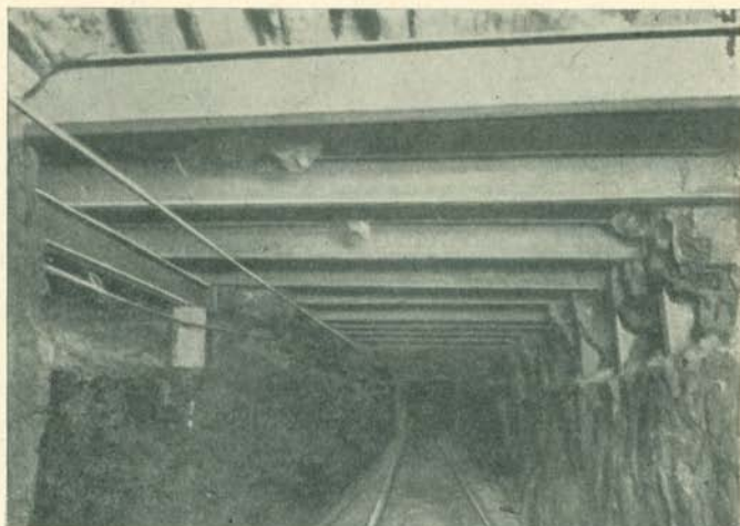
Steel Beams laid on Coal and Short Posts
