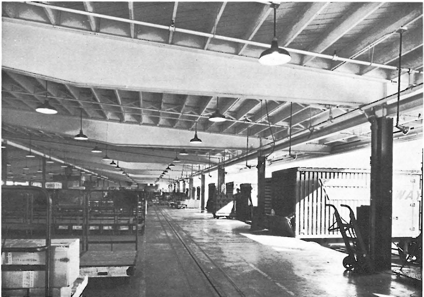
Consolidated Freightways Transfer Depot—Los Angeles, Calif. Stiles & Robert Clement, Architects-Engineers Note cantilever support for roof over loading platform
