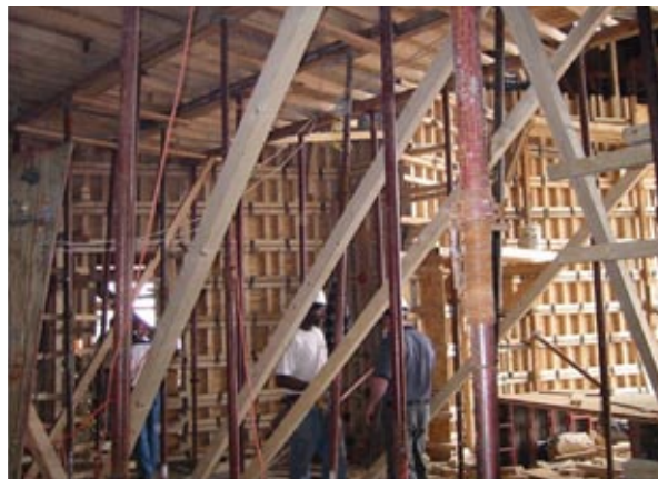
Shoring creates waste in concrete projects.
