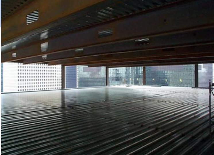
Long spans and open vistas with steel mean less waste is created.
