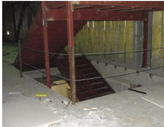
Steel is adaptable for future building renovations.
