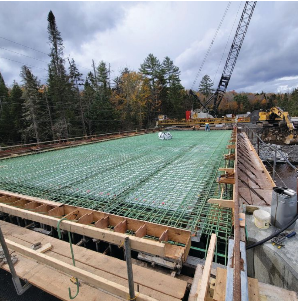
above: Stay-in-place steel deck forms were installed on the new bridge.
