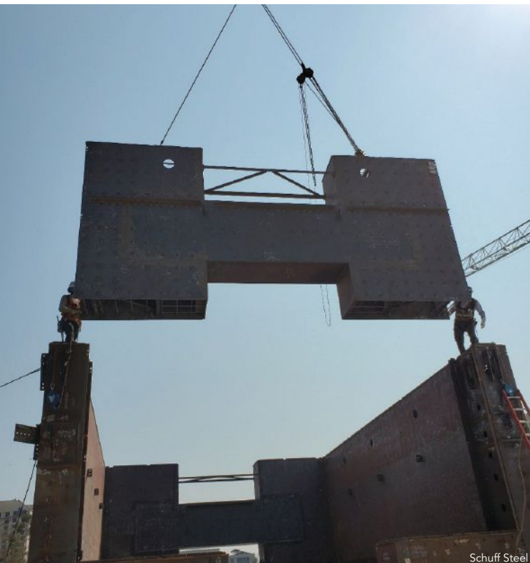
left: Prefabricated SpeedCore pieces being erected.
