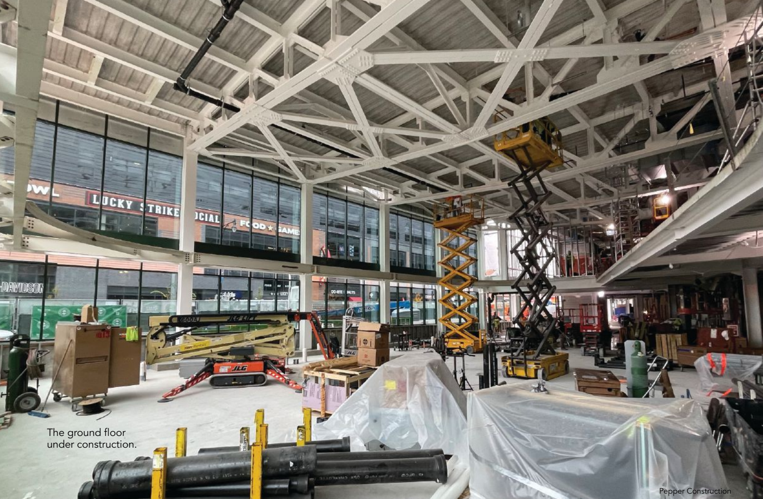
The sportsbook interior with the cantilevered balcony and roof trusses.
