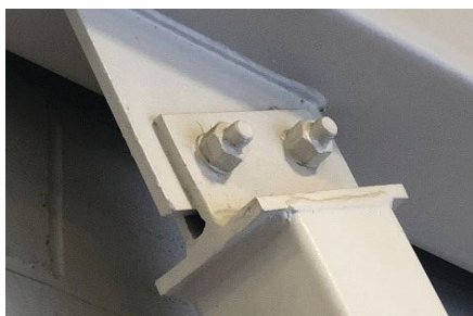
Fig. 8. End tee connection, with two stems, to a square HSS bracing member.
