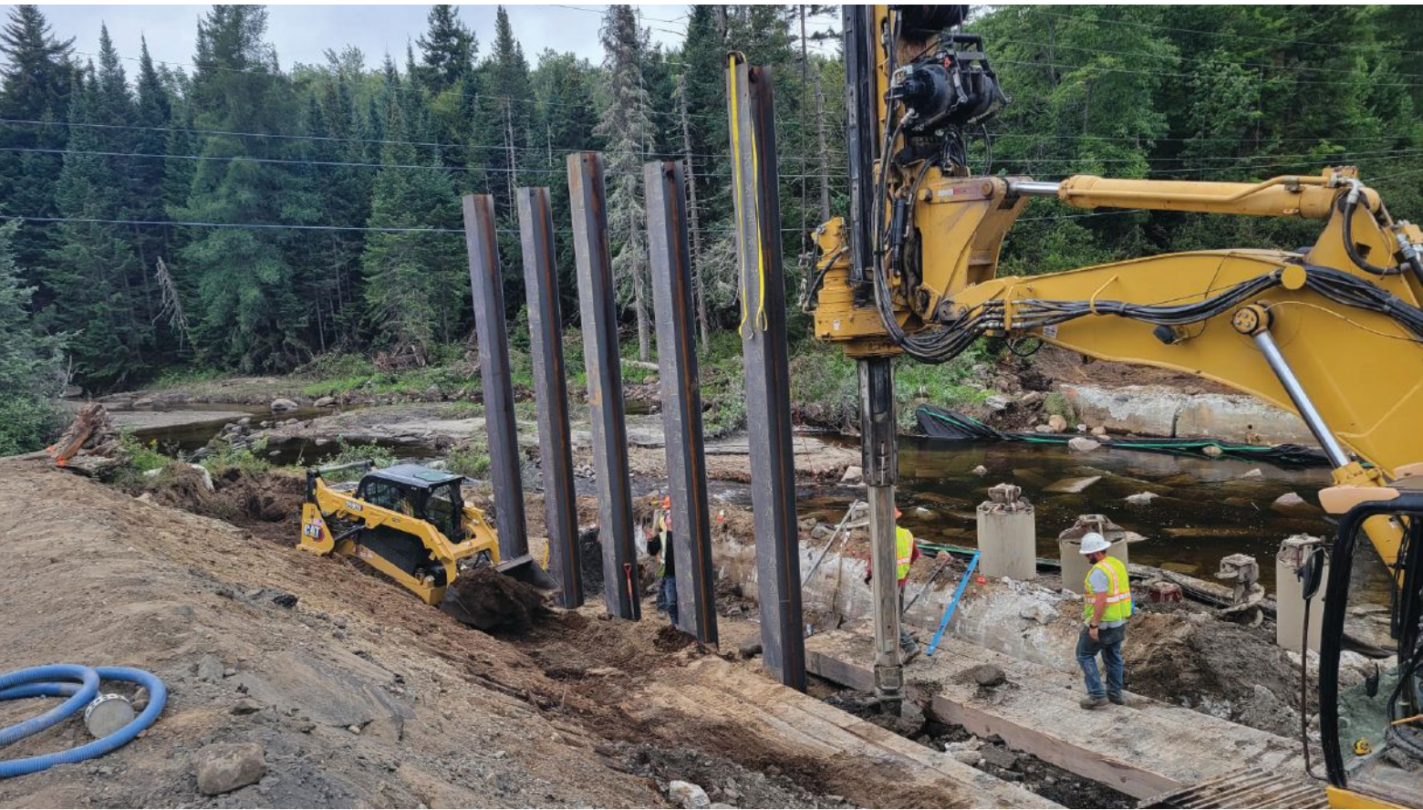
above: Steel H-piles being installed at new abutment locations.
