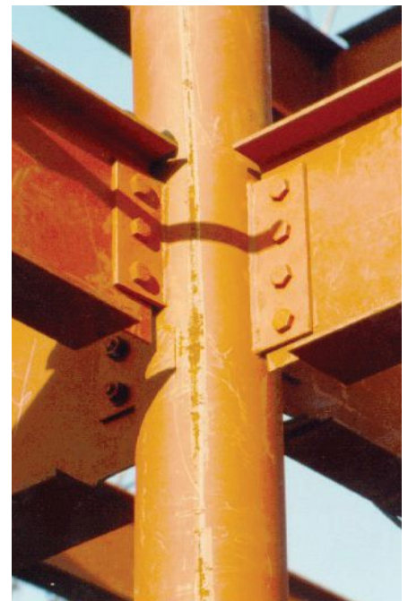
Fig. 6. Single-plate shear connection to round HSS column.
