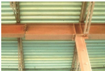
Fig. 7. Continuous beam over a square HSS column.
