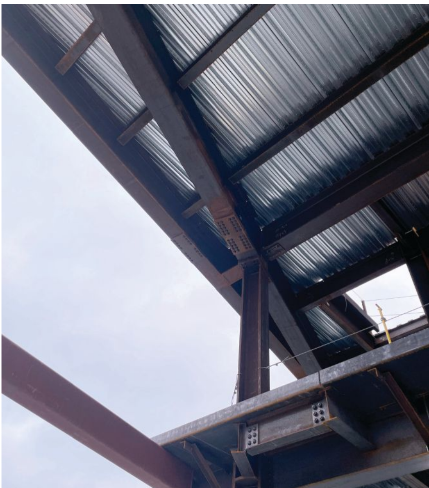
A closer look at one of the W36x487 backspan girders.
