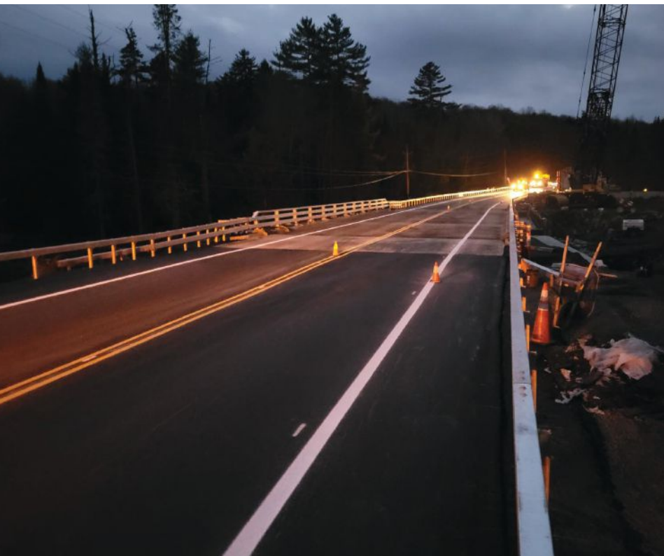
below: The new bridge opened to traffic on October 27.
