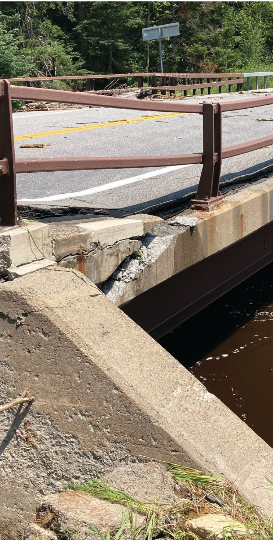
A close-up look at the damage a July 2023 flood inflicted on the State Route 28N bridge over Fishing Brook.
