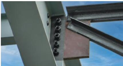
Flush-frame connection designed for efficiency
