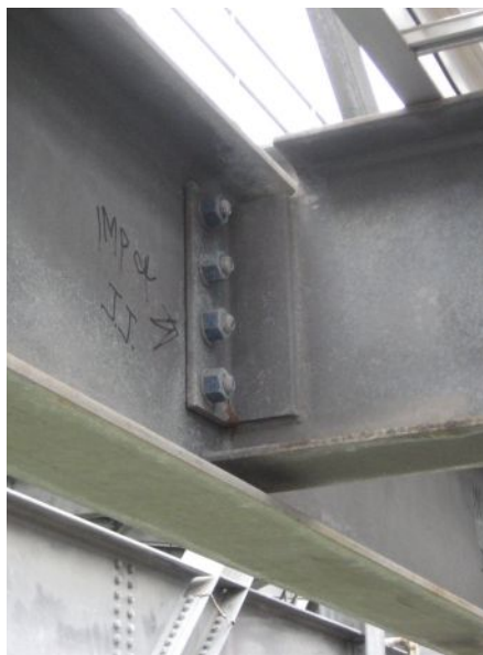
a. Heavy industrial structure Fig. 6. Single-coped beams.
