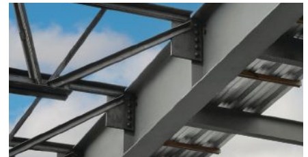
Joist reaction point occurs at beam centerline
