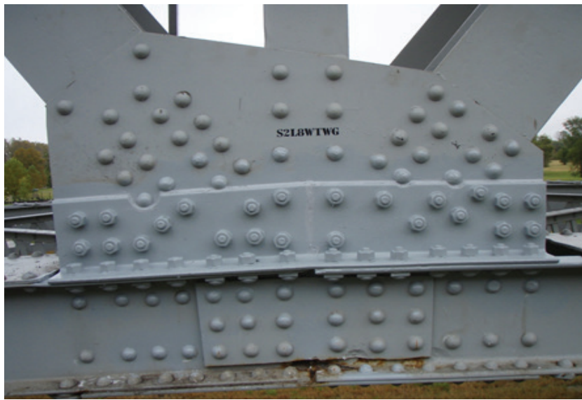
Figure 3-25—Final repair installation after sealing contact surfaces and application of topcoat
