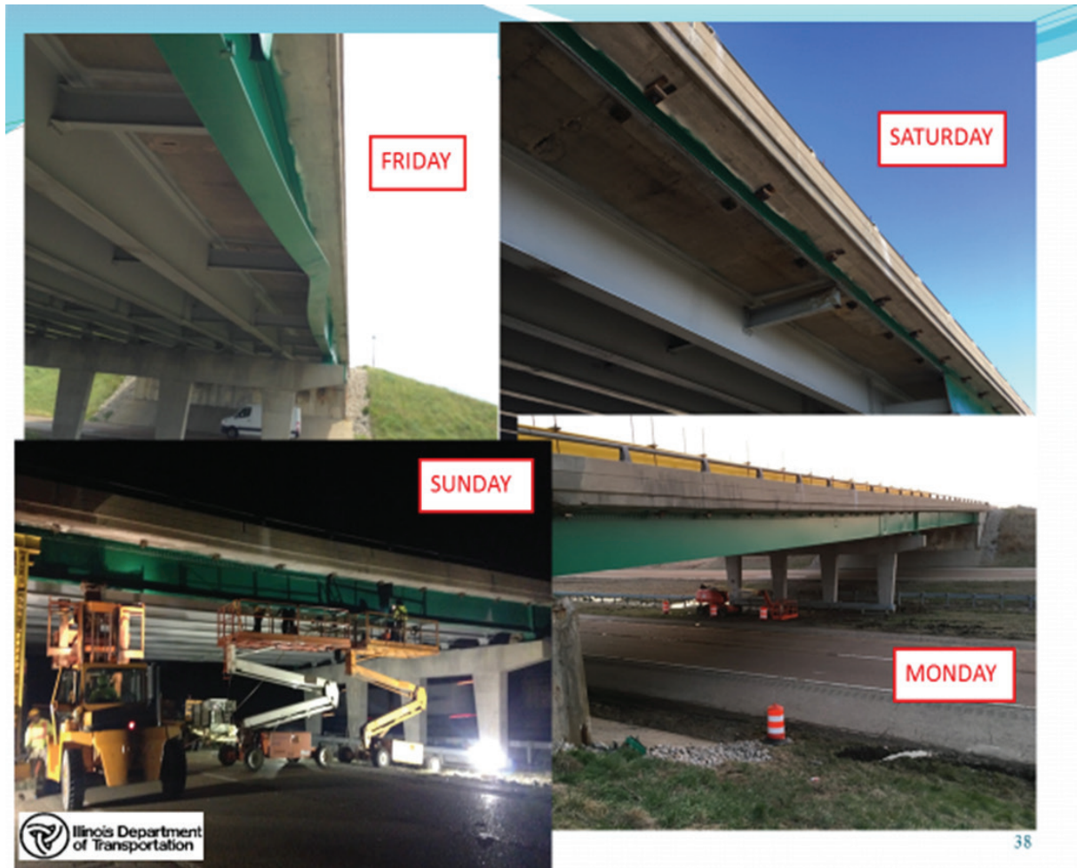
Figure 5-13—Photos illustrating primary stages of partial beam replacement (Illinois DOT)
