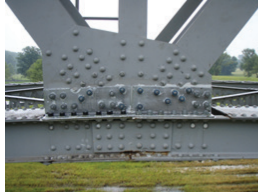
Figure 3-24—Installing steel repair and tightening bolts
