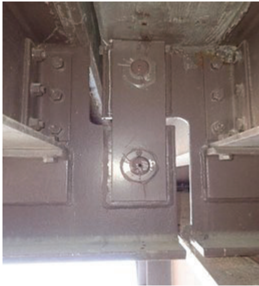
(a) Pin and hanger with exposed pins
