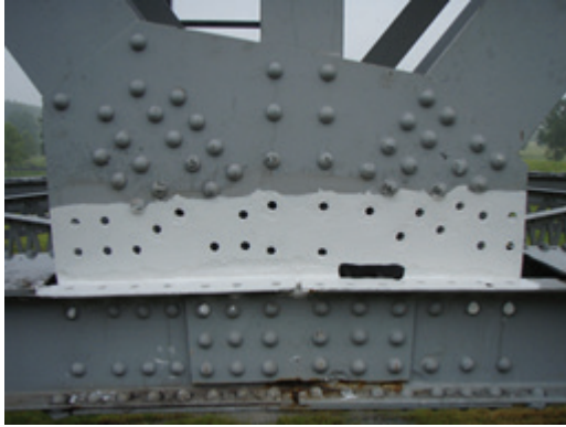
Figure 3-23—Coating exposed steel surfaces
