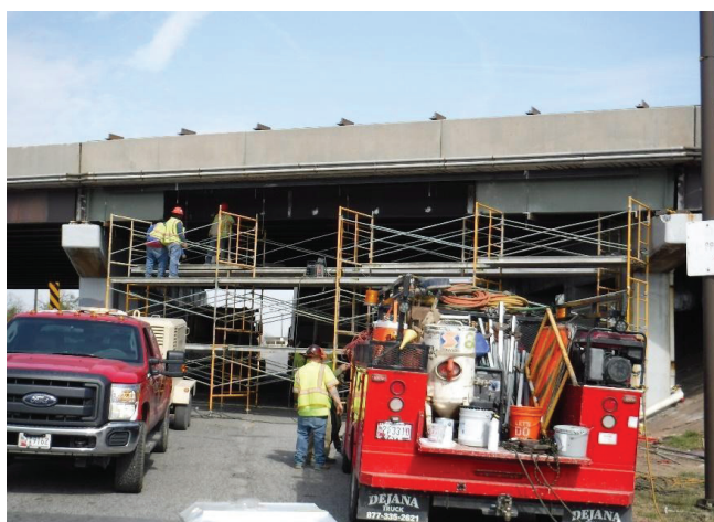
Figure 5-7—Full-Depth Removal (Maryland Transportation Authority)
