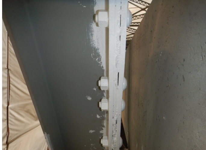
Figure 3-10—Plating repair where epoxy filler hardened prior to plate installation
