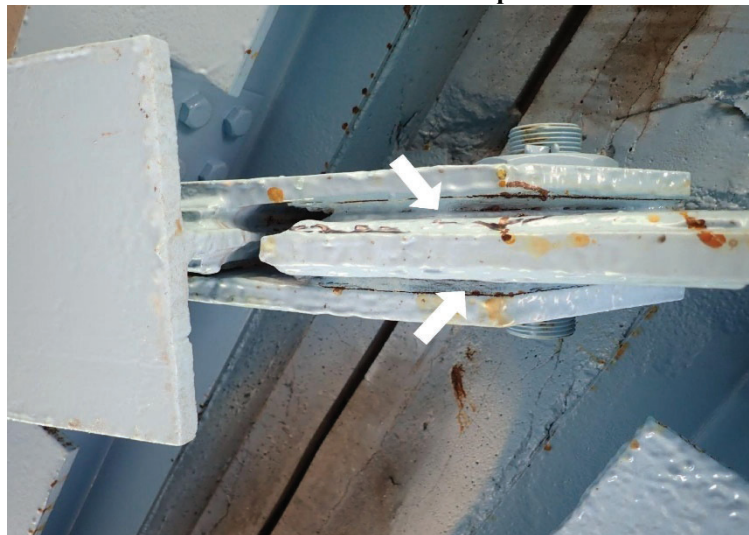
Figure 3-46—Pack rust between the pin plates (arrows) that creates unintended tensile stress in the pin
