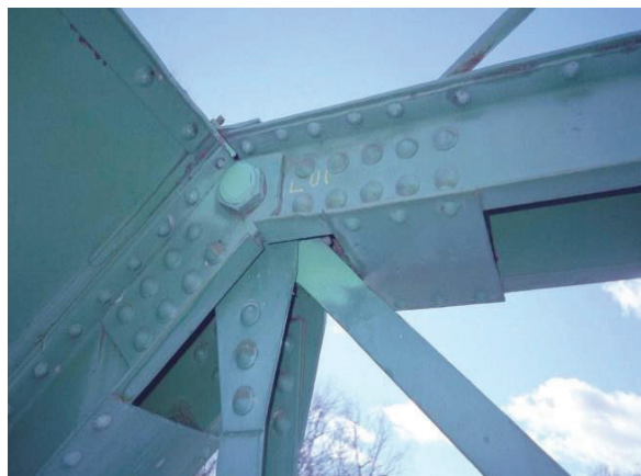
(b) Pin-connected truss members
