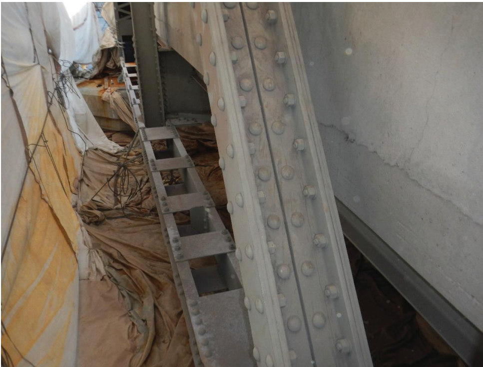
Figure 3-4—Photo of plating an existing W-shape with built-up angles
