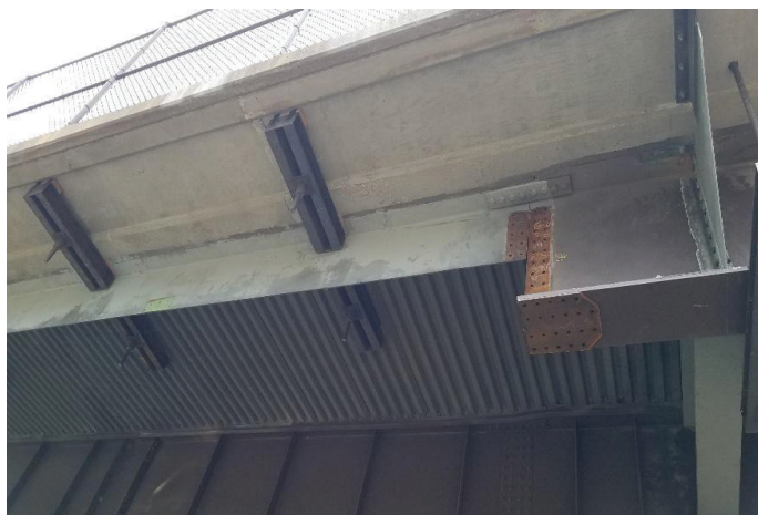
Figure 5-6—Partial-Depth Removal (Maryland Transportation Authority)
