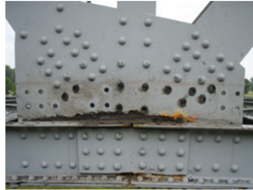
Figure 3-21—Holes drilled on existing gusset plate
