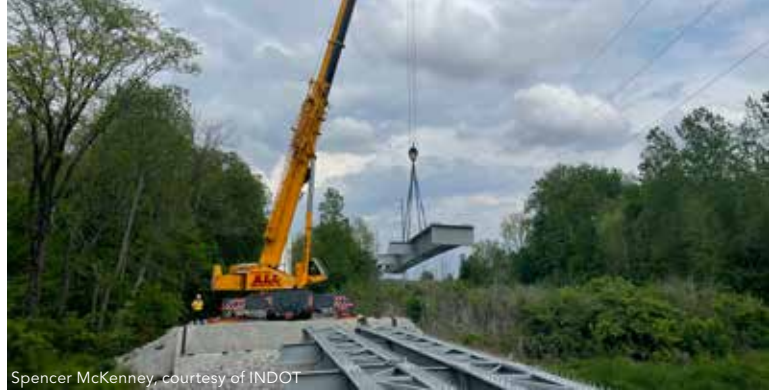
Spencer McKenney, courtesy of INDOT
