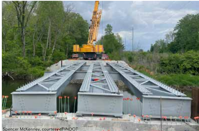
Spencer McKenney, courtesy of INDOT
