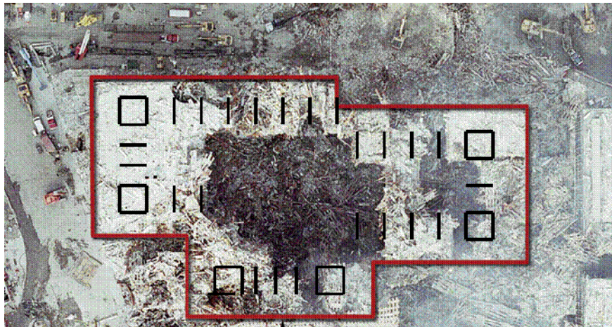
Figure 5. Collapse of World Trade Center 6, induced by falling debris from the North Tower. Note that the dark lines indicate approximate locations of one-bay steel moment frames around the building perimeter.
