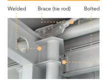
Lateral, tension, and compression forces must travel from beams, braces, and columns down to foundations through connections.
