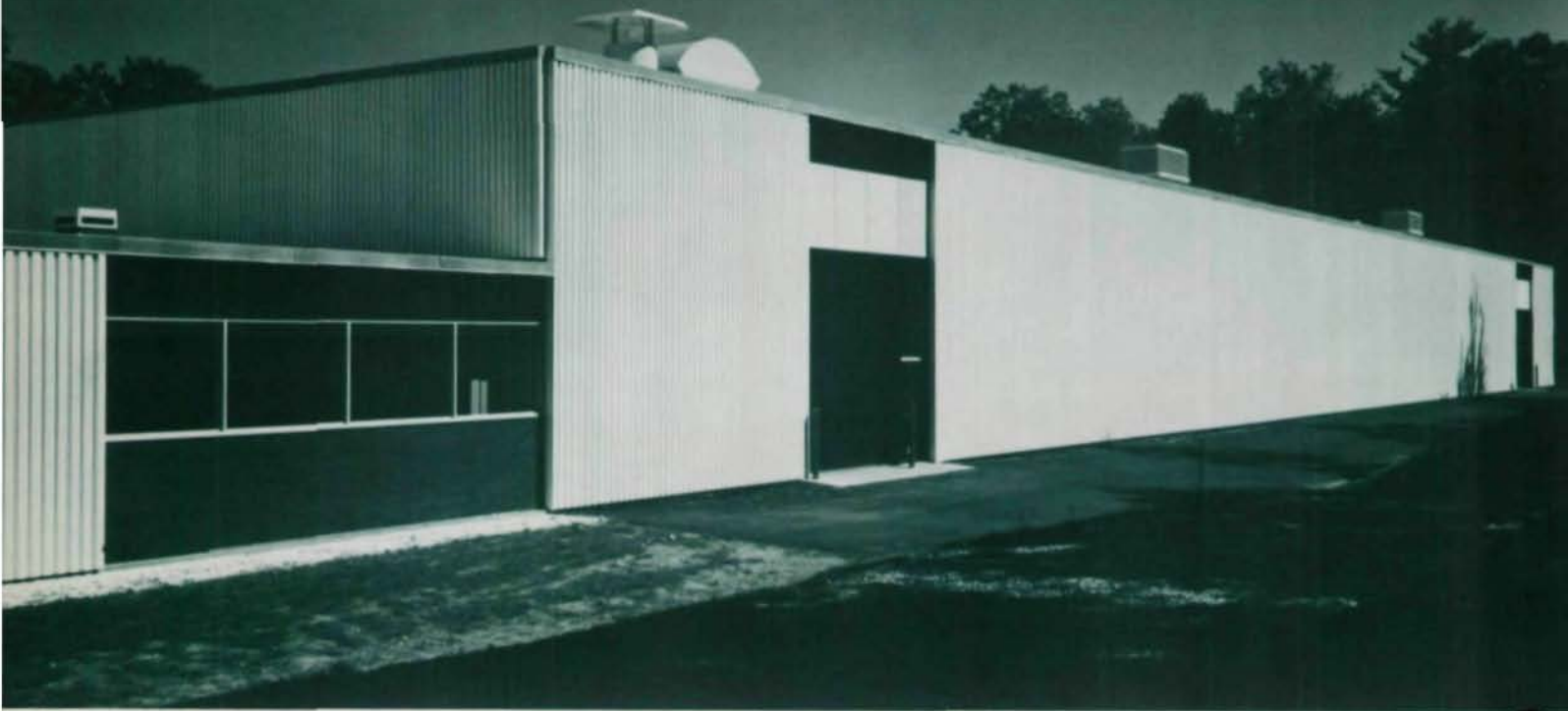
Structural Steel Framing Facilitates 72,000 sq ft expansion.
