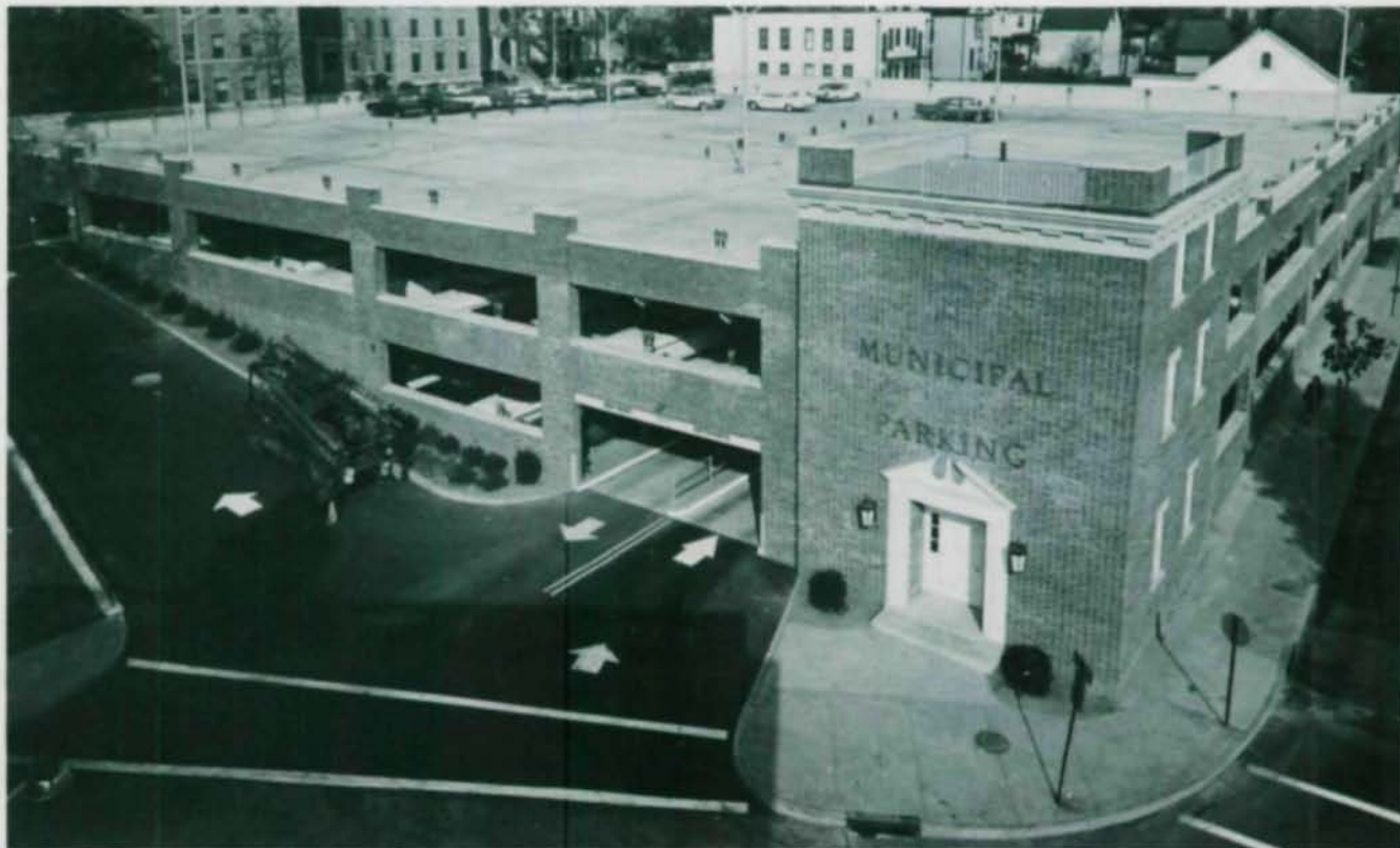
Based on using new AISC specification and high strength steels past cost studies were reevaluated. Result - steel framing was selected and a trend was reversed.
