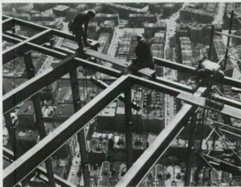
Topping-out nears as ironworkers swing final steel into place.
