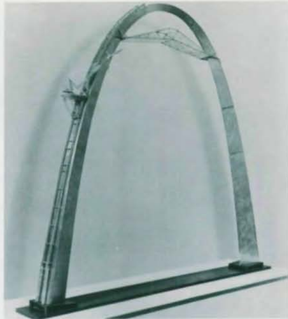
Model shows how crane with 100-foot boom will ride 42-by-32-foot platform up each leg to lift huge sections into place. This method was one of several developed by Pittsburgh-Des Moines Steel Company to build the giant stainless steel monument.
