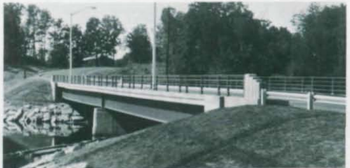
AWARD OF MERIT – SHORT SPAN Bridge Over Moose River, Lyons Falls, New York Designer: New York State Department of Public Works Owner: State of New York Fabricator: Gouverneur Iron Works General Contractor: Thomason & Perry Inc.
