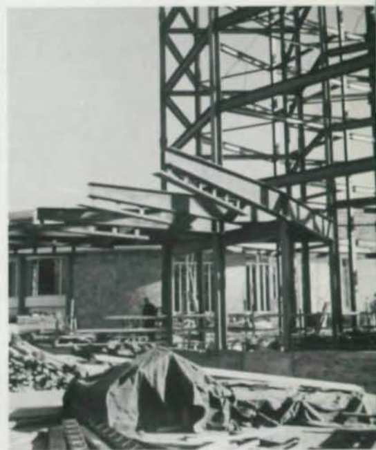
Steel frame was completed in 22 days despite freezing weather. Five tapered girders fan out from single column to frame canopy.
