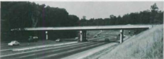
AWARD OF MERIT – HIGHWAY GRADE SEPARATION Linden Lane Over Capital Beltway (I-495), Forest Glen Park, Maryland Designer: Maryland State Roads Commission Owner: Maryland State Roads Commission Fabricator: Atlas Machine & Iron Works General Contractors: Wright Contracting Company G.A. & F.C. Wagman, Inc.
