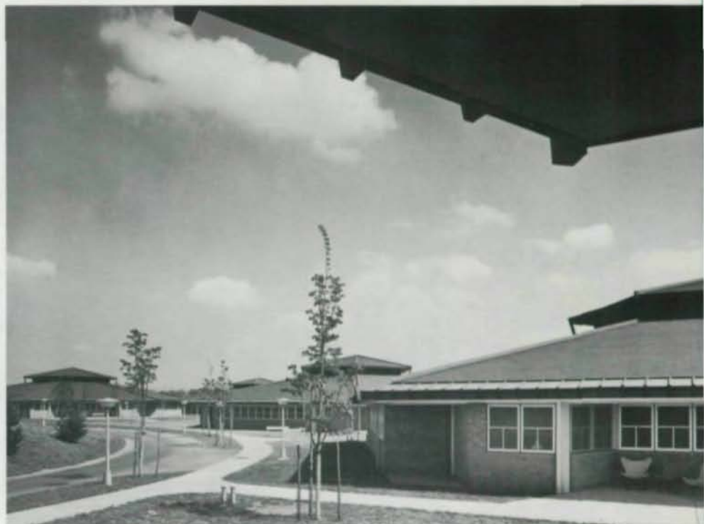
Welded sun sheds were "flipped" in mid-air after being assembled upside-down on ground. High roofs of cottages were also assembled on ground, then lifted on to low roofs.
