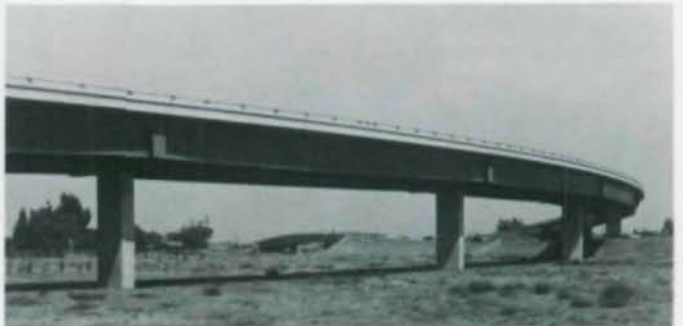
AWARD OF MERIT – HIGHWAY GRADE SEPARATION Northbound Route 280/17 Separation, San Jose, California Designer: State of California Owner: State of California Fabricator: Herrick Iron Works General Contractor: Gibbons & Reed & Dan Caputo
