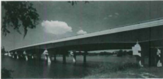
AWARD OF MERIT – MEDIUM SPAN LOW CLEARANCE City Park Lake Bridge, Baton Rouge, Louisiana Designer: Modjeski and Masters Owner: Louisiana Department of Highways Fabricator: American Bridge Division, U.S. Steel Corp. General Contractor: Boh Brothers Construction Company
