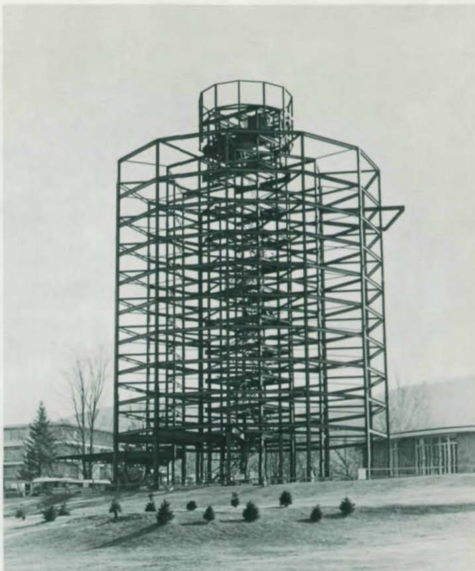
Steel frame was completed in 22 days despite freezing weather. Five tapered girders fan out from single column to frame canopy.
