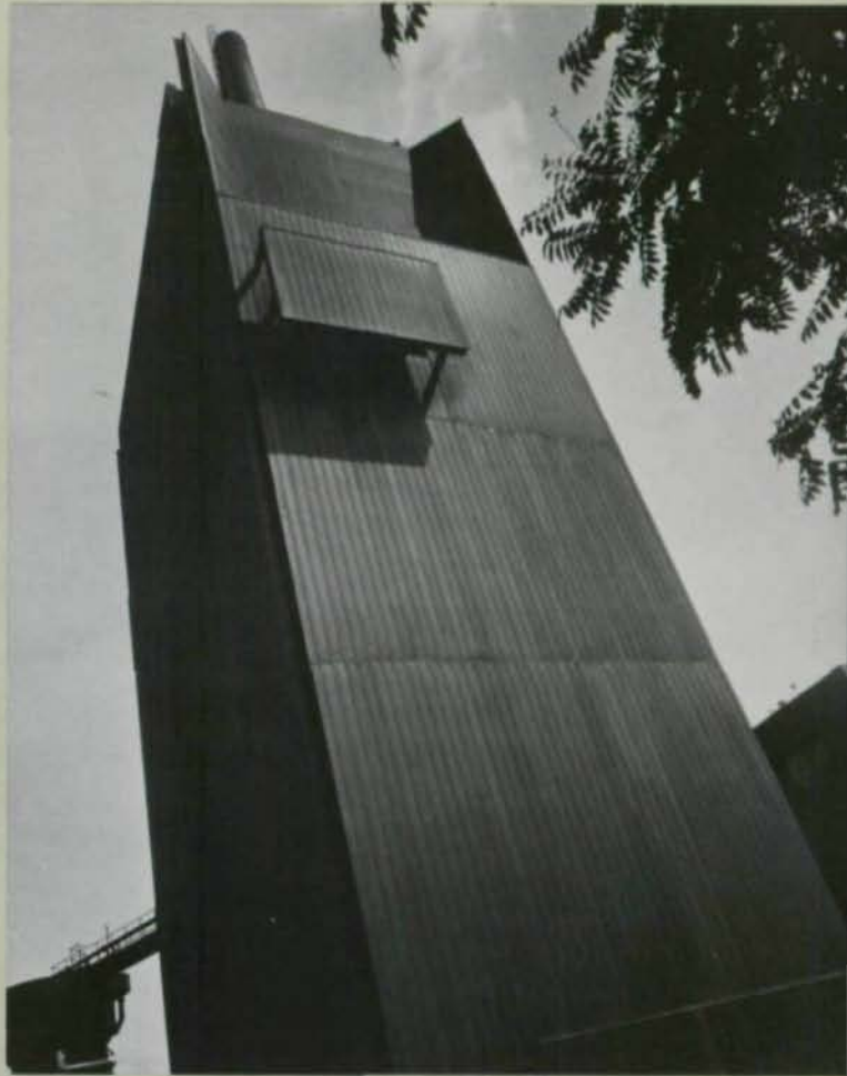
▲ BOILER PLANT ADDITION Terre Haute, Indiana Architect: Archonics Corporation
