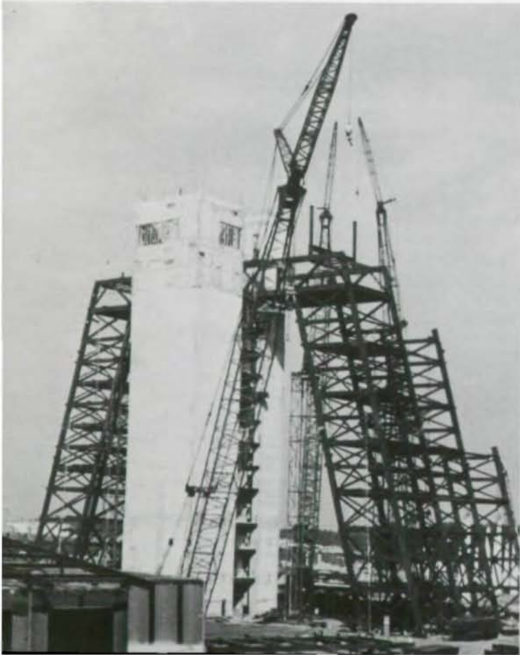
Thirteen pairs of 150-ft high steel A-frames were erected around a central elevator core.
