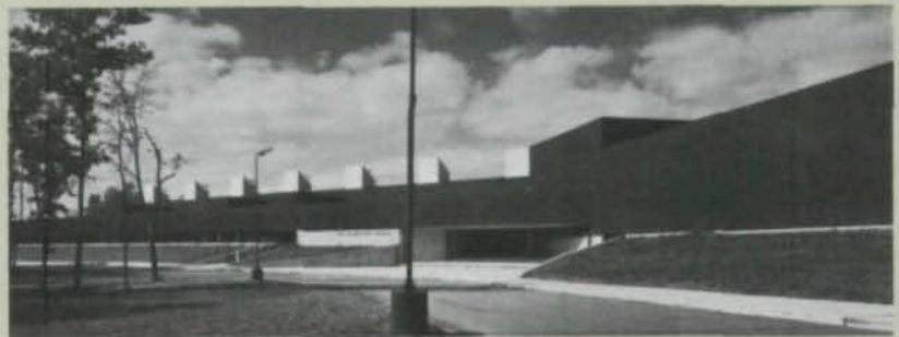
MONGUAGON SCHOOL Trenton, Michigan Architect: Eberle M. Smith Associates, Inc.
