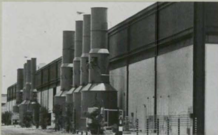
▲ AIRCRAFT ACCESSORIES OVERHAUL SHOP (P-108) (P-110) San Diego, California Architect: Daniel, Mann, Johnson, & Mendenhall
