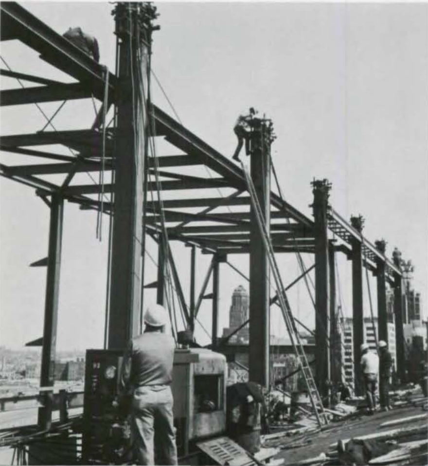
Extended steel columns support the lifting jacks.
