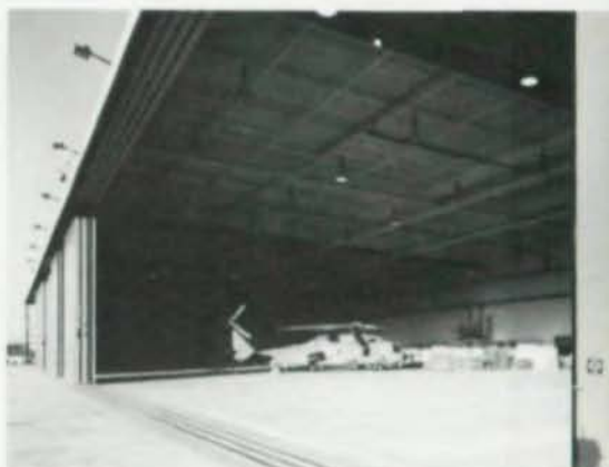
Operational side of North Island hangar
