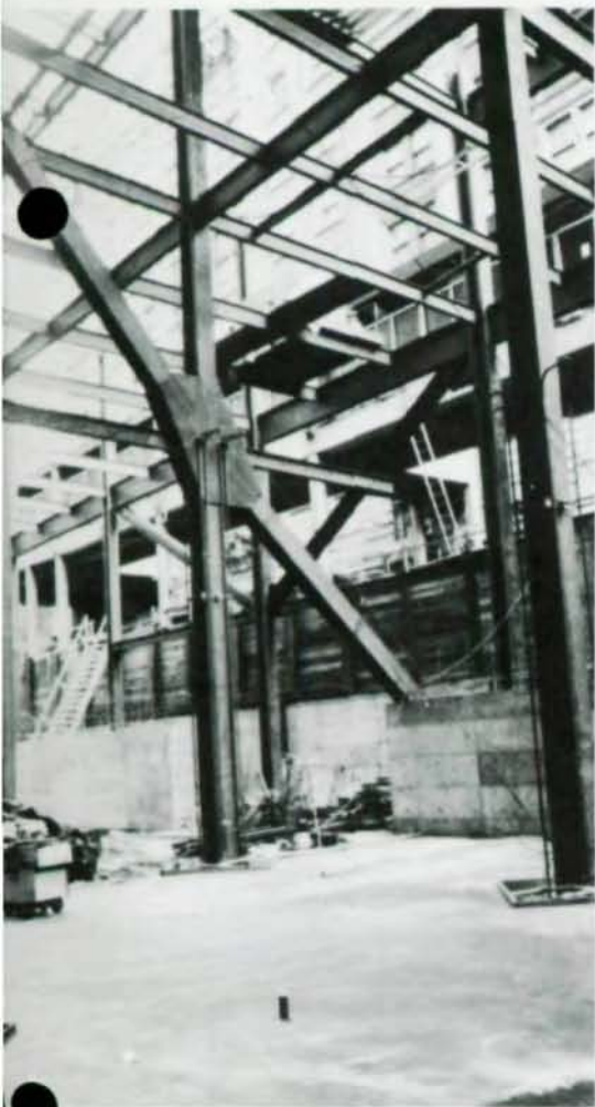
All bracing connections are field-bolted, with gusset plates shop-welded to columns (l.). Typical bracing detail (Fig. 3, above). Photos by David McCullough and THP Limited.
