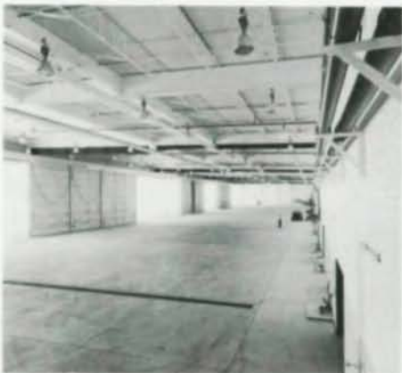
Hangar bay showing steel trusses
