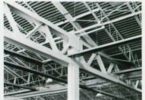
Nine airlines share Lambert air cargo complex (l.). Structure's versatility comes with 25-ft modular steel-framed construction, adapted to each carrier's needs (below, l. & above).
