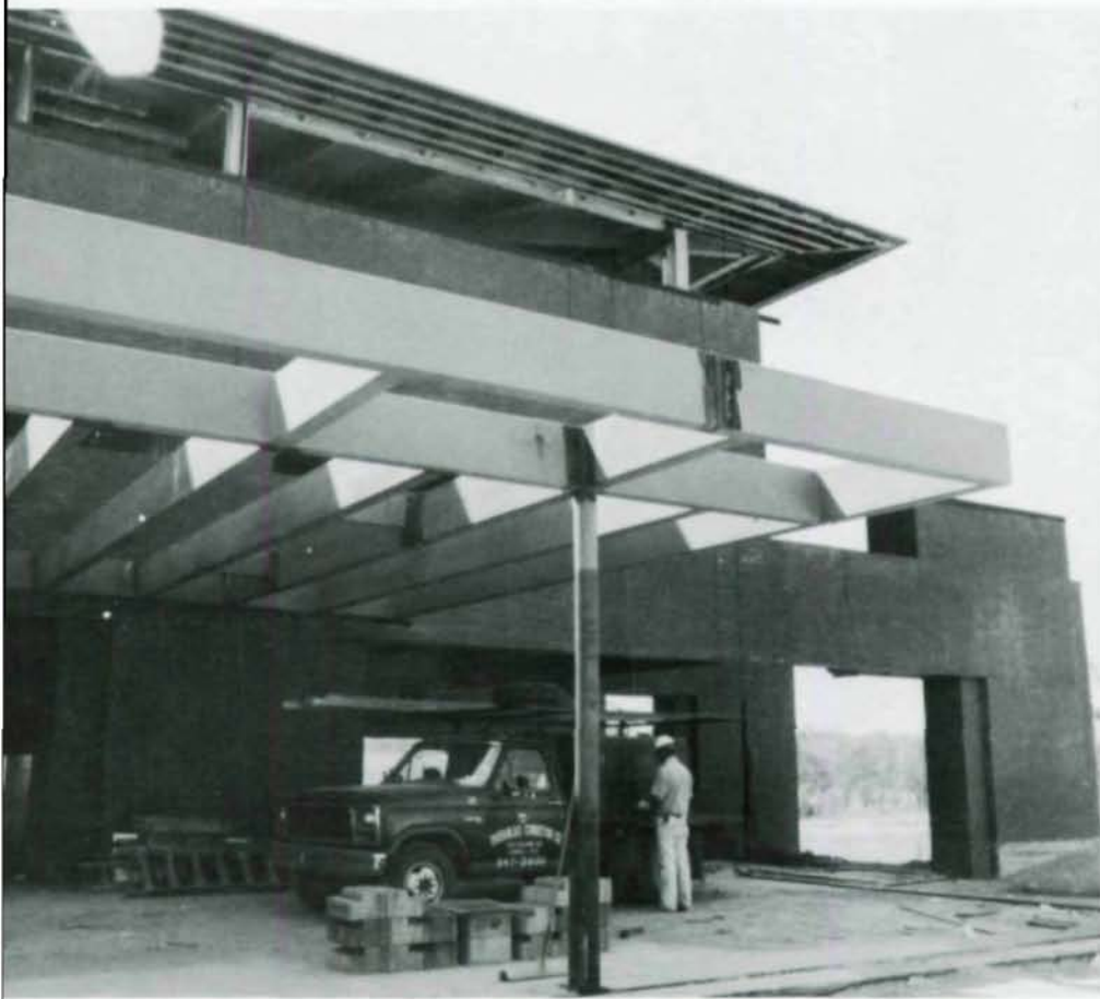
Steel-frame supported trellis carries through on Wright design.
