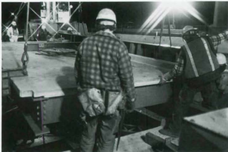
New sidewalk section is set in place. Photos by D. Siemans.
