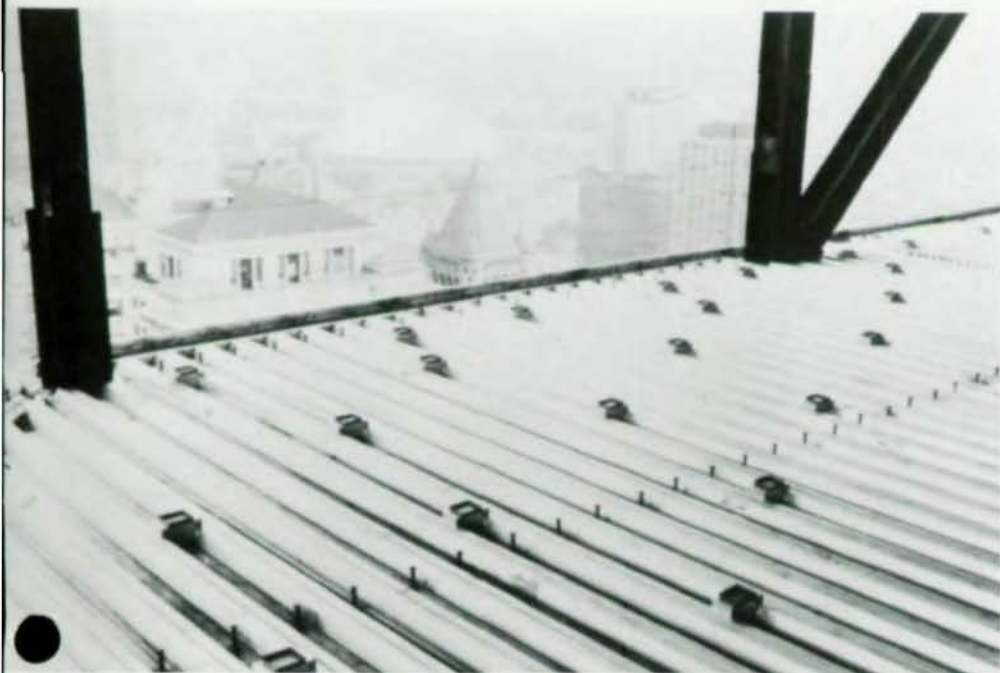
According to steel industry, two essentials that keep an intelligent building up-to-date and adaptable are structural steel framing and electrified flooring (l. and above). The tunnel-like raceways hold wiring and fiber optics that control systems and services. Central switching system (r.) is fully digital, capable of voice and data transmission simultaneously.
