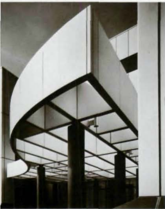
Handsome entry (l.) is steel-framed. Lateral seismic and wind loads resisted by K-bracing in exterior walls (below). Three-cell metal deck (bott., r.) with preset inserts provides adequate power outlets.
