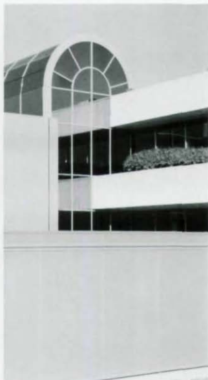
Curving glass vaults rise over walkways, set off in their own environment (l.). Exterior (r.) shows steel curtain wall which resulted in 60% savings.
