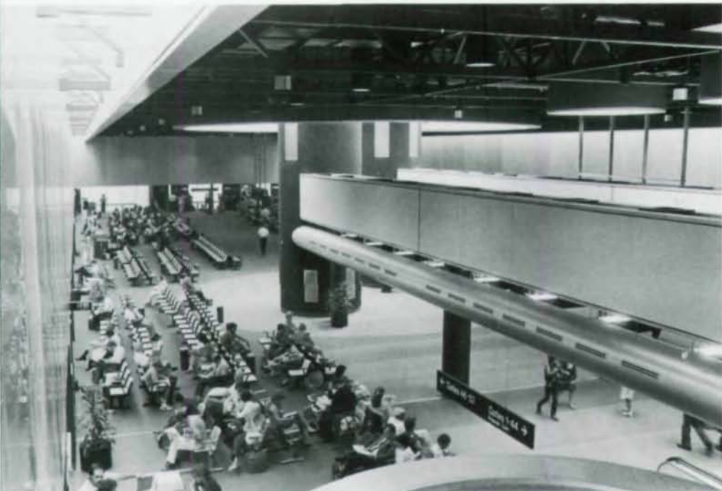
Spacious quality achieved by architectural interaction of exposed steel trusses and skylighting in 2-story rises of TWA concourse.
