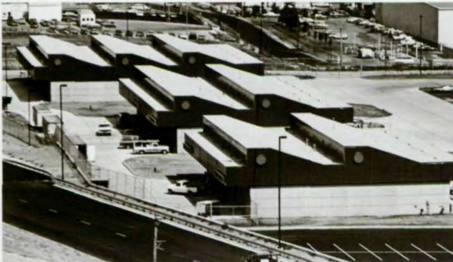
Nine airlines share Lambert air cargo complex (l.). Structure's versatility comes with 25-ft modular steel-framed construction, adapted to each carrier's needs (below, l. & above).
