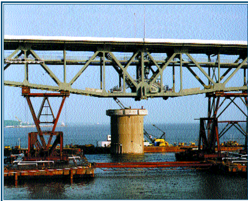
Fig. 3. Span of Coleman Bridge supported by unique barge-tower transport system. Tower design required innovative steel connections described in article.
