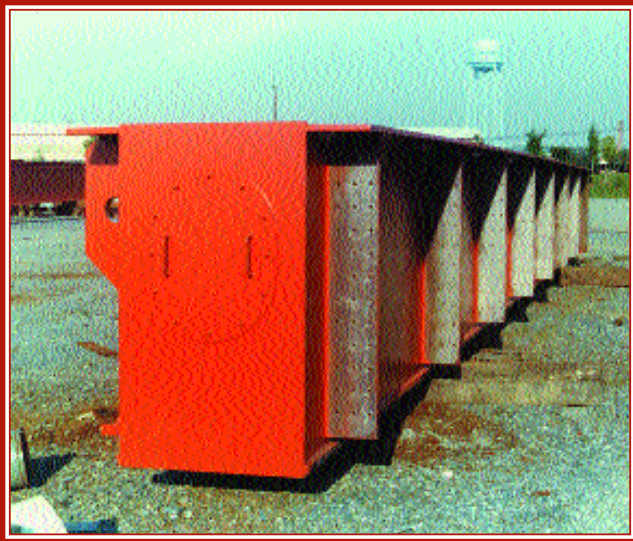
The proper placement and proper size of access holes is very important in box girder design
