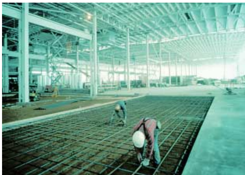
The installation of production area flooring. Photo courtesy of Clark Construction.
