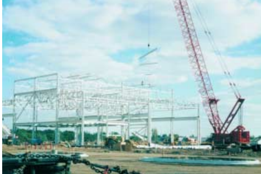
The facility's specifications outlined the use of hot-dipped galvanizing on all exposed steel.
