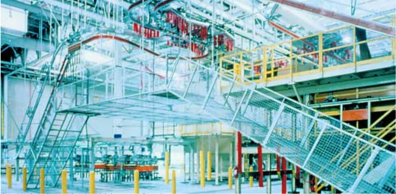
Interior view showcasing the high bay manufacturing area.
