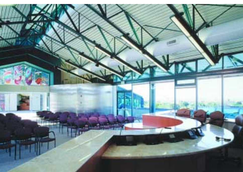
Exposed steel joists and girders are on display at the 3 rd floor council chamber.
