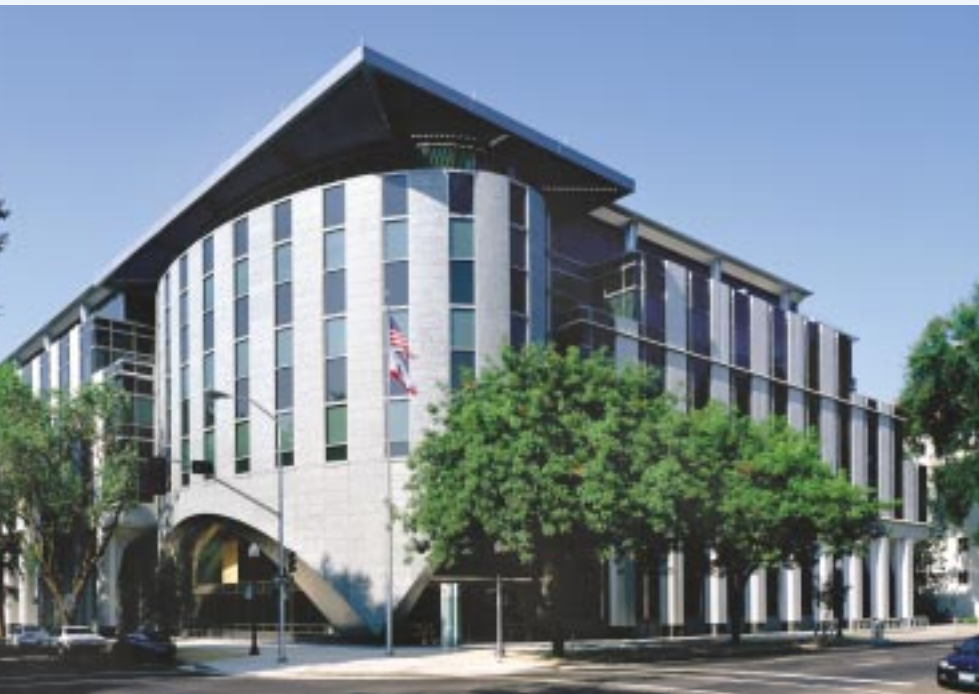
The elliptical shape of the front lobby extends up through four stories.
