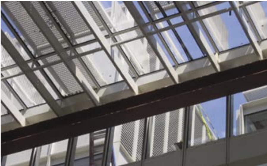
Portion of completed skylight at the Piazza.
