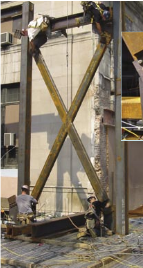
Diagonal bracing at the "Cube" during erection. (Photos by Frank Prial, Beyer Blinder Belle)
