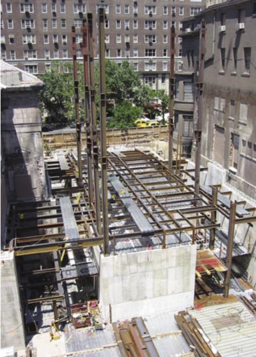
Far Left: Rock excavation below street level.
