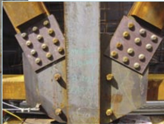
Diagonal bracing at the "Cube" during erection. (Photos by Frank Prial, Beyer Blinder Belle)
