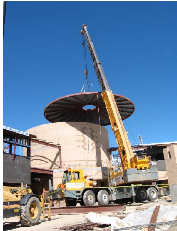
The circular rotunda roof, using HSS8x4x¼ joist members framing into HSS10x4x¼ tension and compression rings, was assembled on the ground and installed as a unit.
