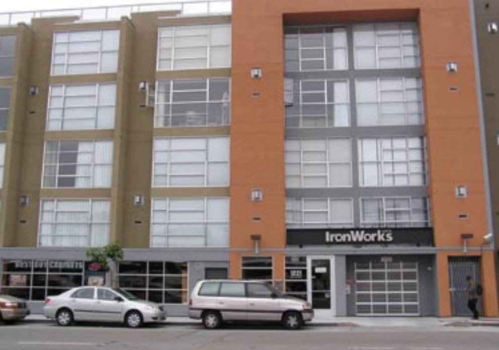
This loft condominium project in San Francisco (also pictured under construction on the previous page) was the first structure to use the Pueblo modular framing system.
