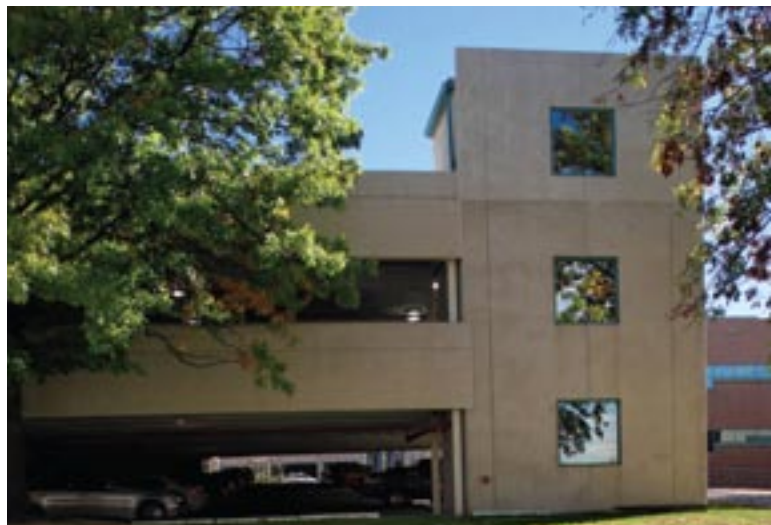
The expansion to the garage added 105 parking spaces.
