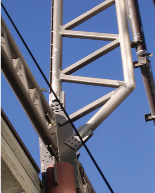
Complex truss connections are featured throughout the building.
