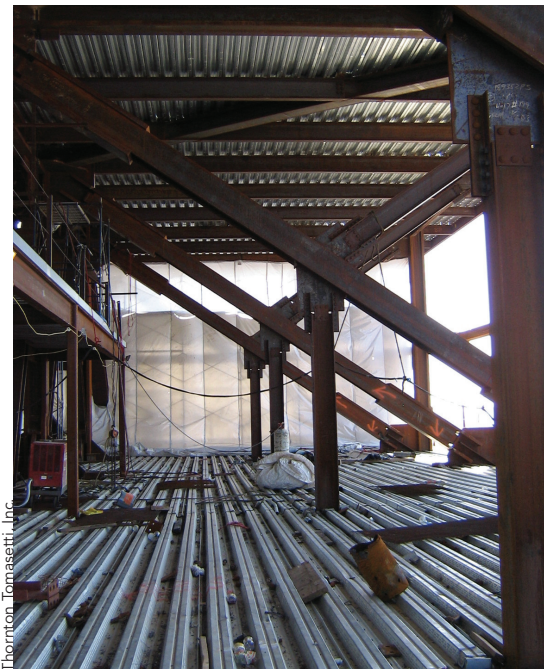
above: Outrigger diagonal braces on the 28th floor.
