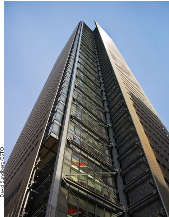
below: Structural elements are brought outside of the building envelope at the four corner notches of the tower.
