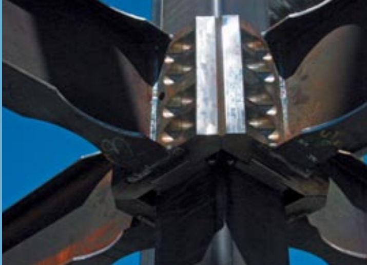
The bolted collars in this assembly were shop-welded via robotics—24 in. of full-penetration welds and 64 in. of fillet welds.
