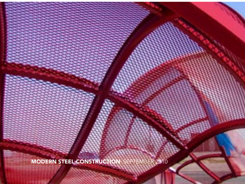
Below: Each piece of wing consists of several expanded metal sections, which required that workers be careful when welding it to the structural members to avoid damage from excessive heat.
