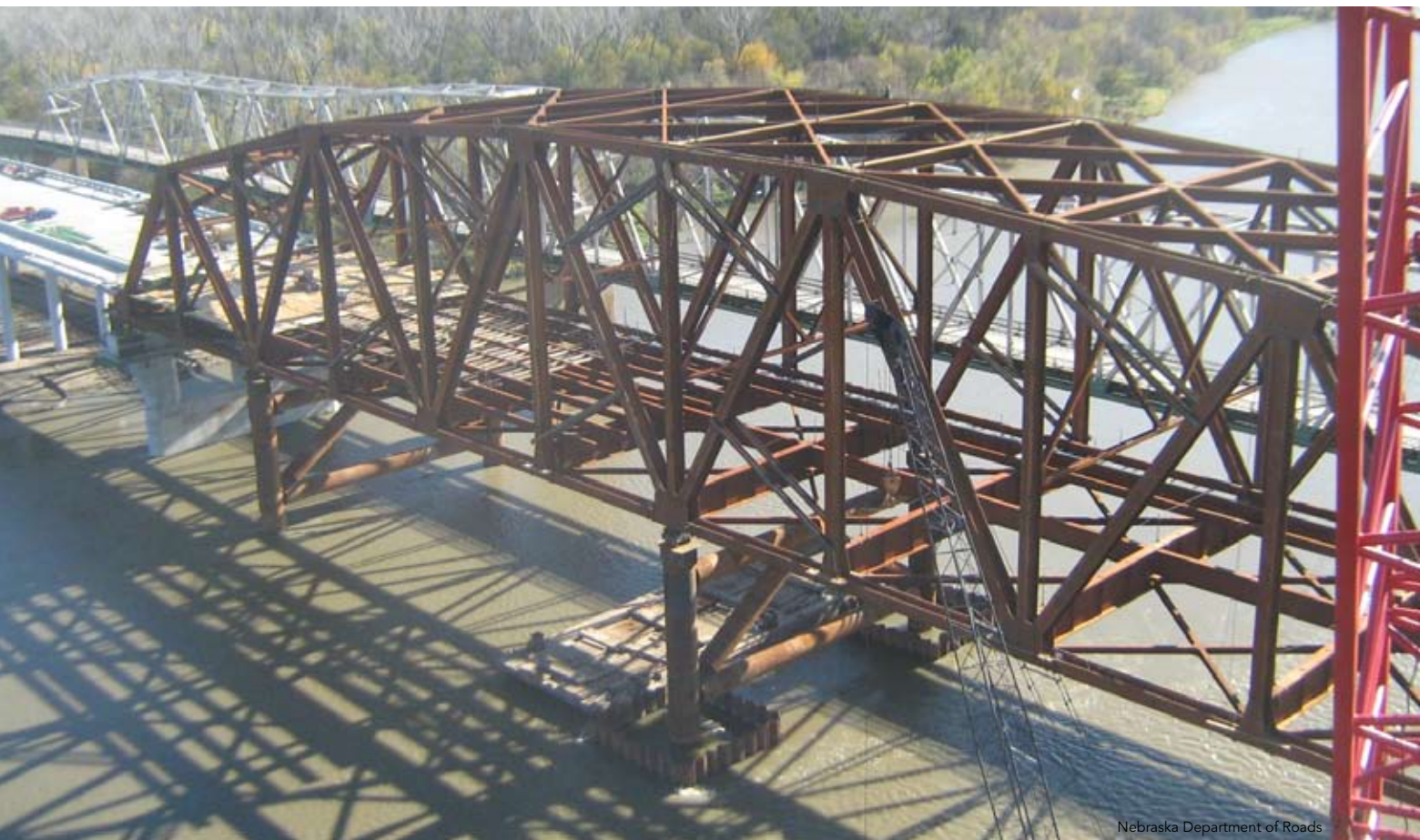
▲ Erection of the Veterans Memorial Bridge utilized temporary bents at L2' and L6.
