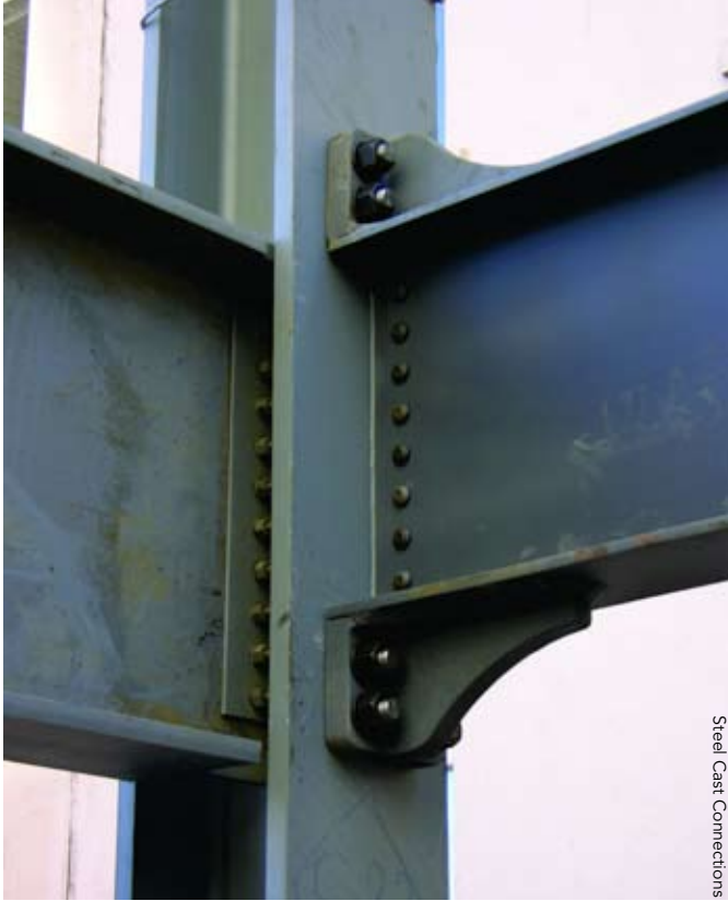
◀ ▲ Kaiser Bolted Bracket connection, W-series.
