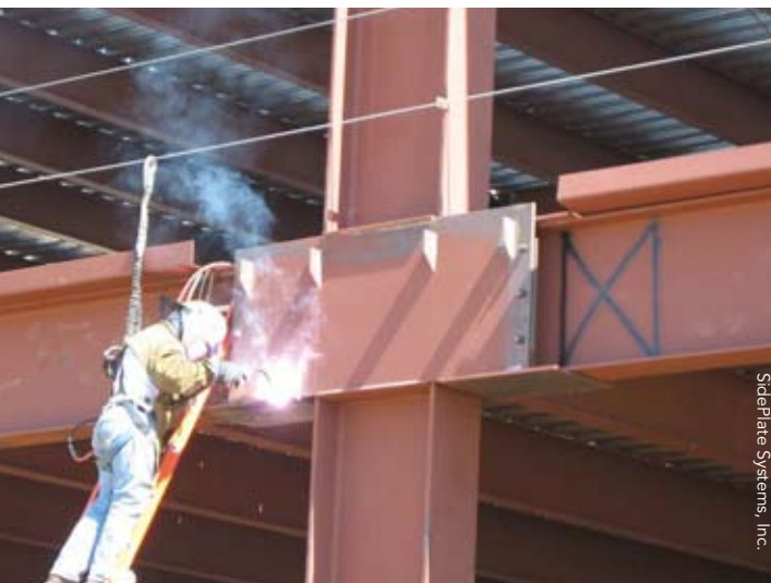
▶▶ SidePlate Frame Connection.
