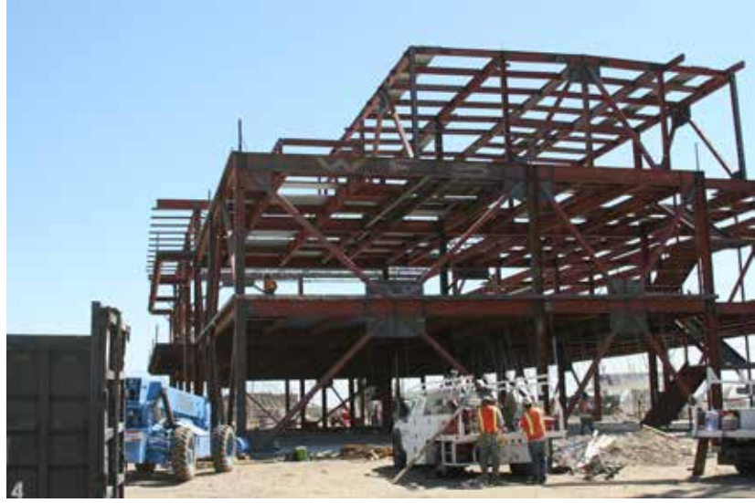
▲ Steel framing allowed for long clear spans in the control room.
