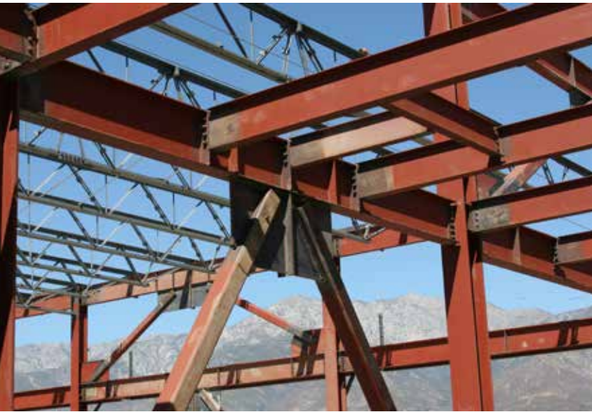
▲ Steel framing allowed for long clear spans in the control room.
