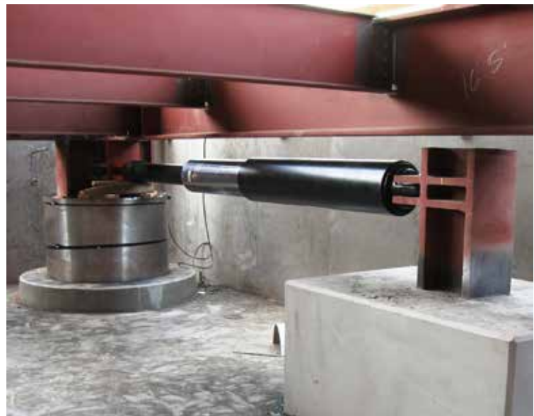
▲ A base isolator with a viscous fluid damper.
