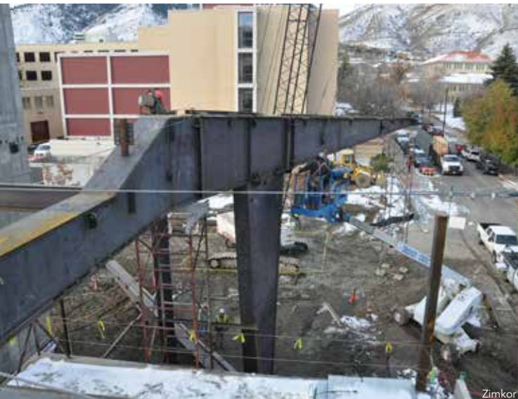
▲ The facility uses 773 tons of steel in all.
