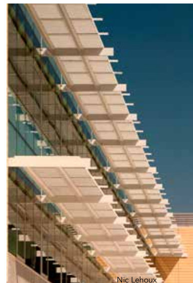
▲ Steel sunshades on the south end of the building.
