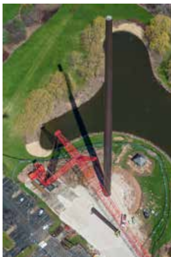
▼ The structure consists of six tubular flanged sections.
