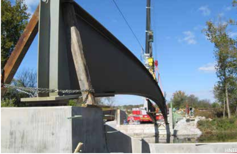
▲ The bridges are composed of haunched welded steel plate girders fabricated from M270 Grade 50W weathering steel.
