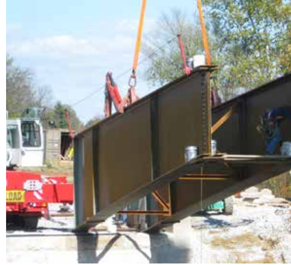
▲ A second girder following the first one.
