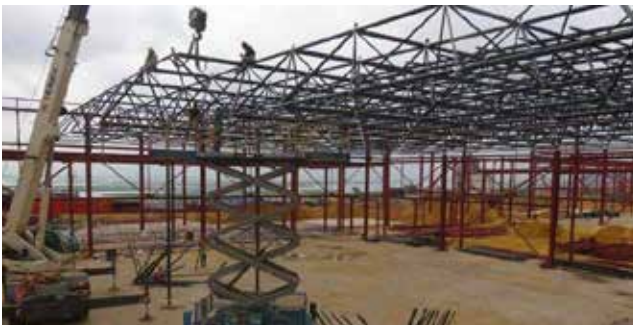
◀ Erection of roofing assemblies.
