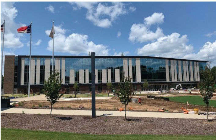
above and below: The new building incorporates more than 300 tons of structural steel in all.
