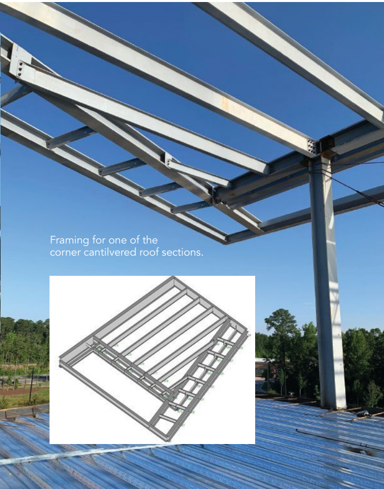
above and right: A bolted plate connection around an HSS column.
