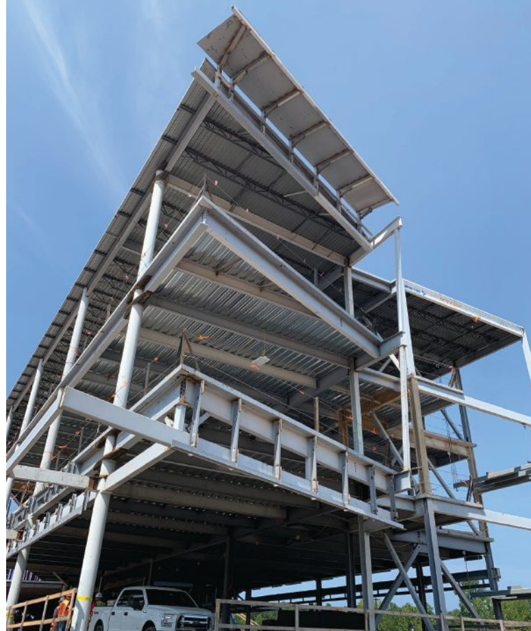
above, below, and right: The two cantilevered ends are clad primarily in glass curtain wall, requiring tight deflection criteria to be maintained throughout the structure.
