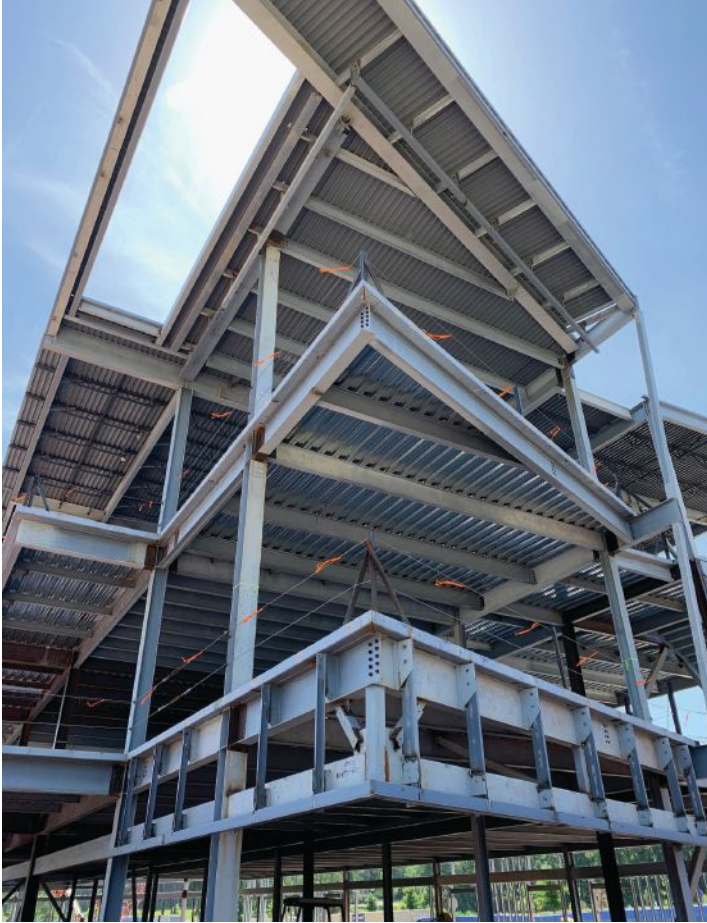
above, left, and right: The three-story structure was designed to cantilever in two different directions at each end of the building.
