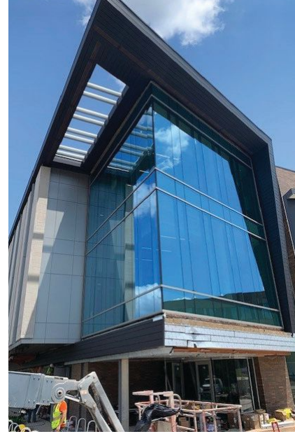
above, left, and right: The three-story structure was designed to cantilever in two different directions at each end of the building.
