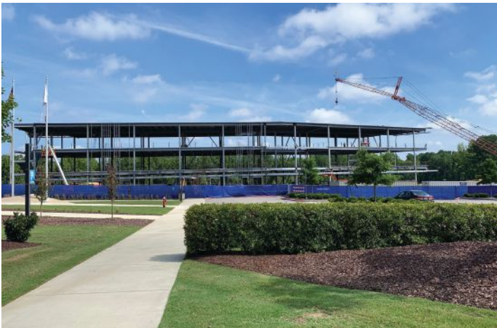
above and below: The new building incorporates more than 300 tons of structural steel in all.
