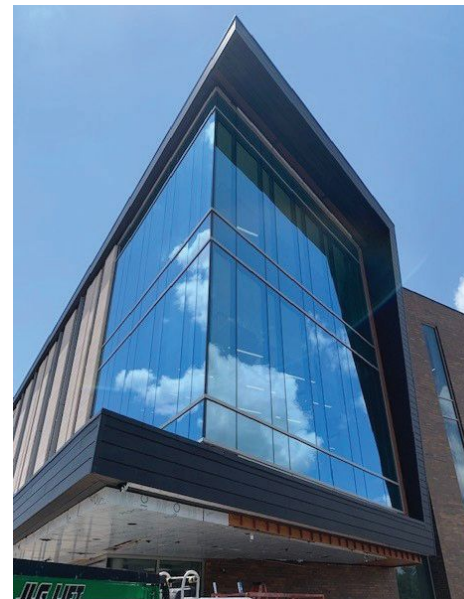
above, below, and right: The two cantilevered ends are clad primarily in glass curtain wall, requiring tight deflection criteria to be maintained throughout the structure.
