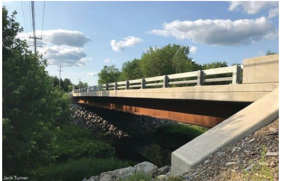
above: The completed Lower Trestle bridge.
