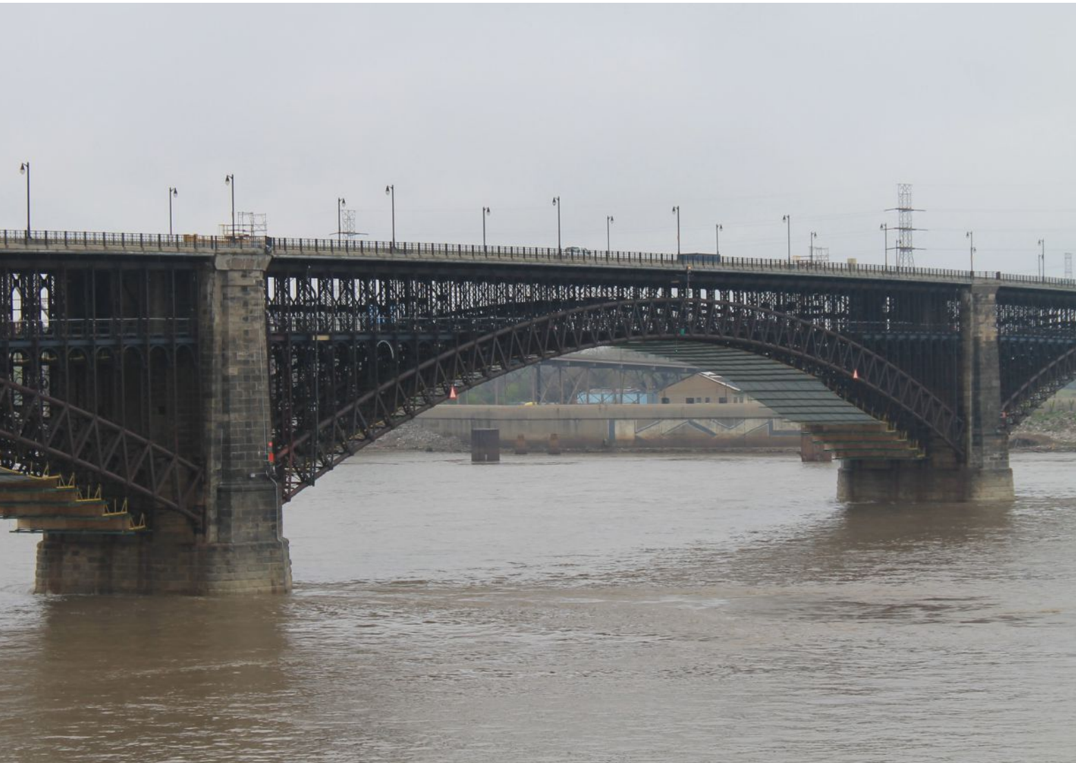
When the Eads Bridge opened in 1874, its 520-ft-long center arch was the longest rigid span ever built. .....
