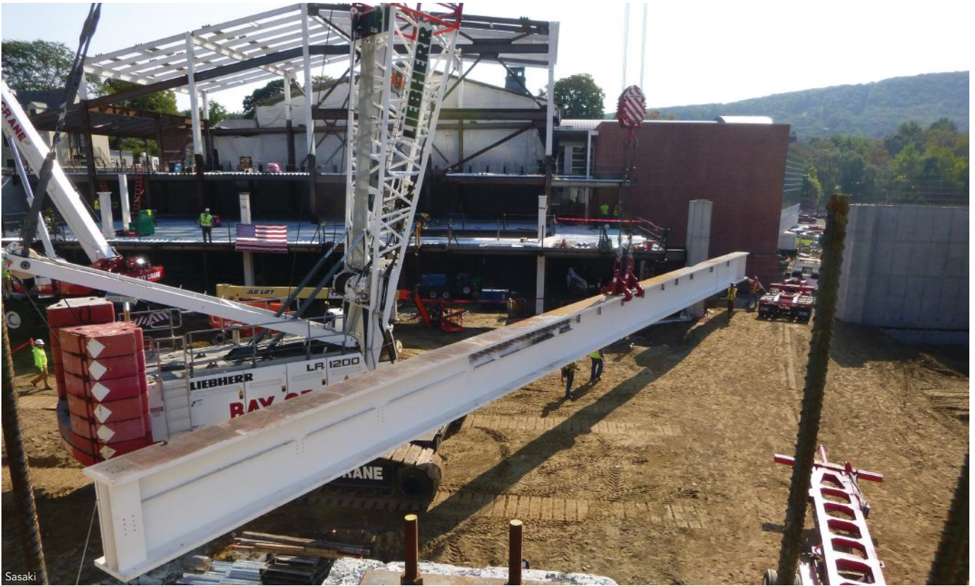
A field House girder and bent with an MEP support truss girder behind it.
