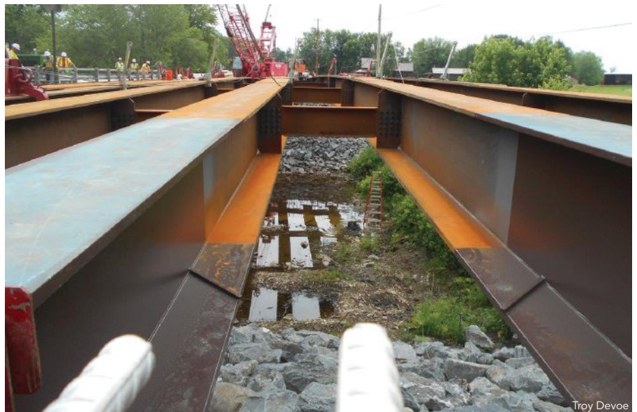
below: Steel plate girder framing for the Lower Trestle bridge.
