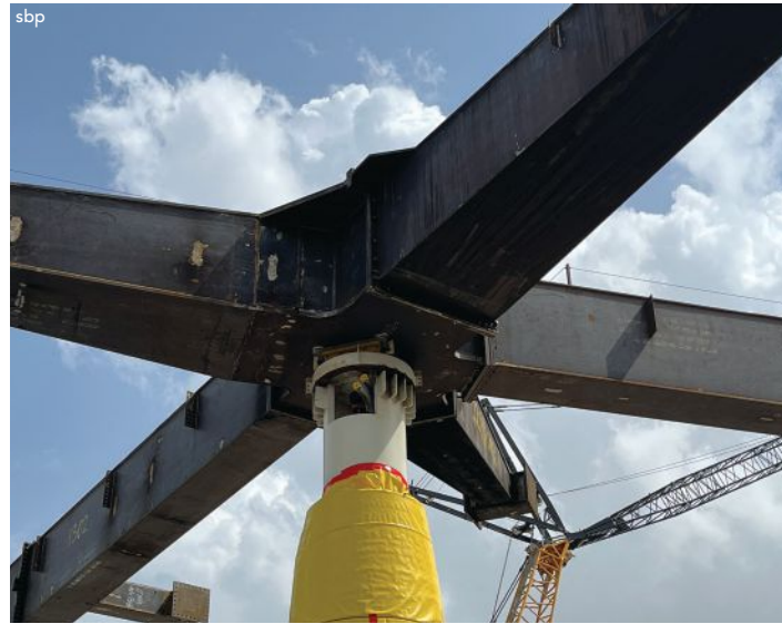
above: The box beam roof girders are laid out like a star.
