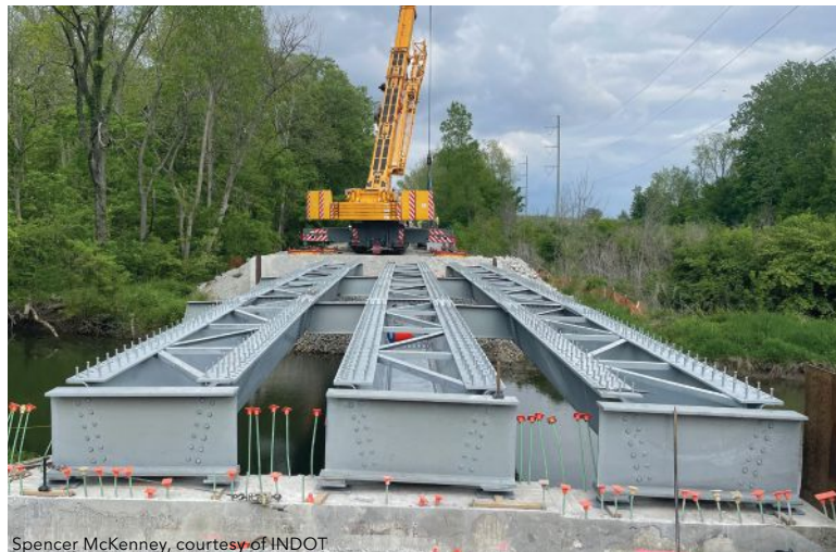
Spencer McKenney, courtesy of INDOT
