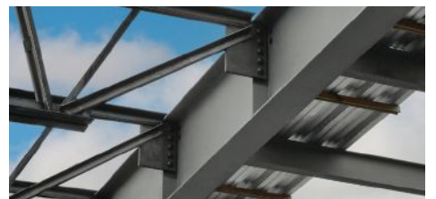
Joist reaction point occurs at beam centerline
