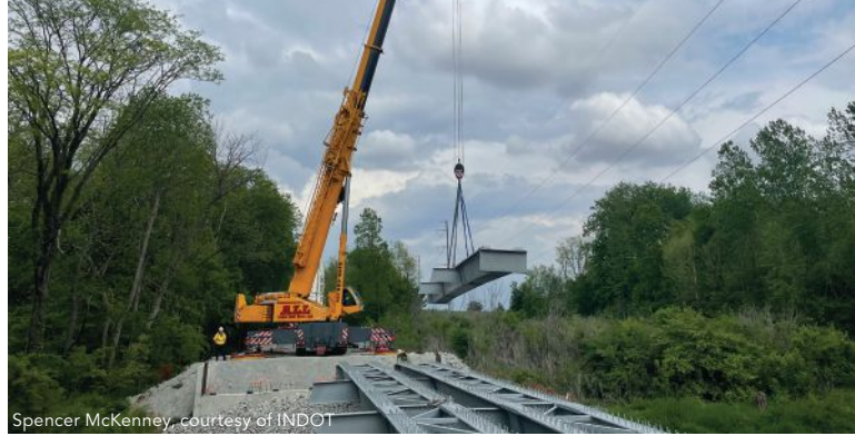
Spencer McKenney, courtesy of INDOT
