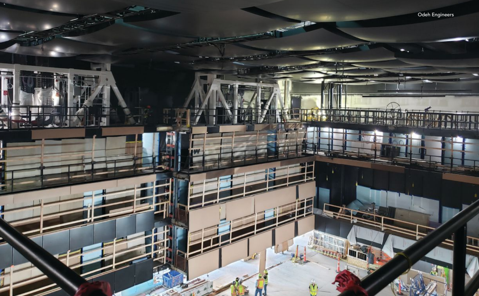
above: The side gantries can move 10½ ft toward the center of the hall, and the rear gantries can move up to 44½ ft toward the stage.
