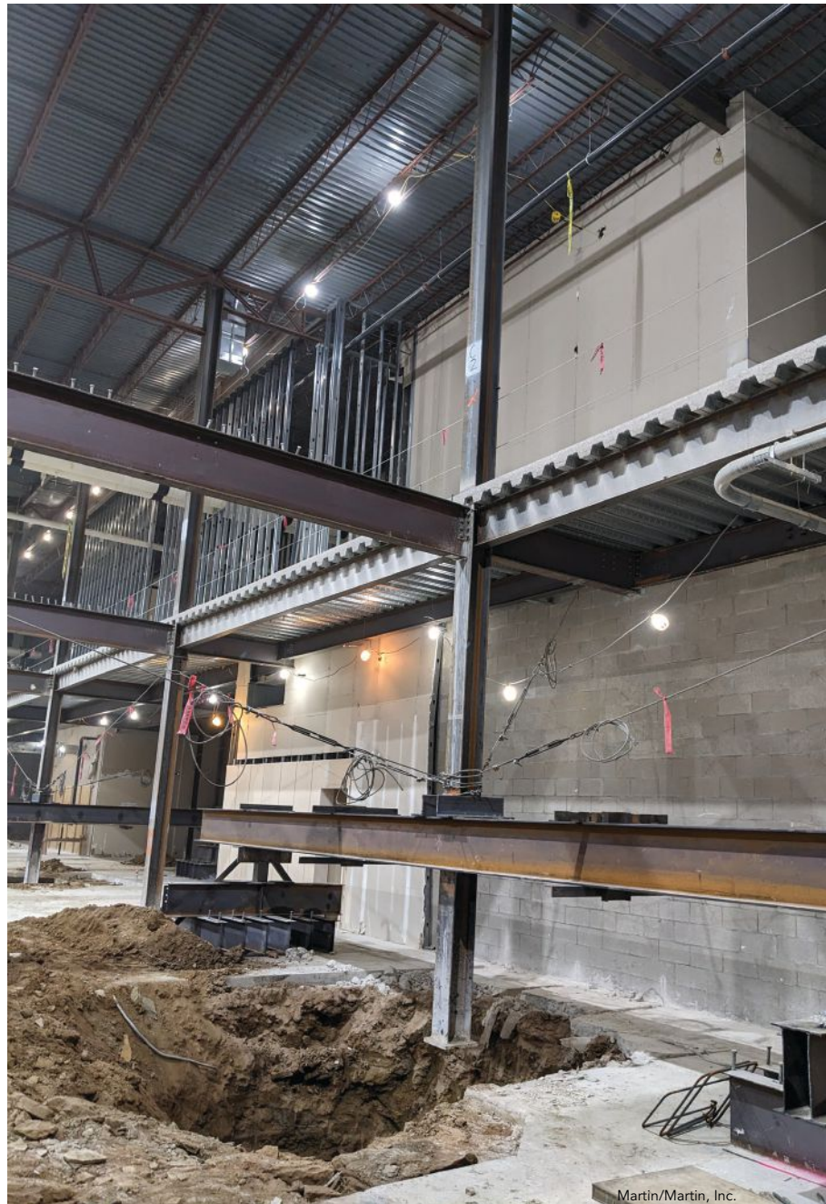
A look at existing steel column shoring during foundation replacement.
