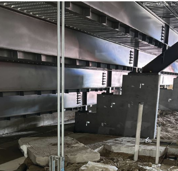
above: The steel-framed raker and seating units. left: Another look at the seating area framing. below: The completed arena interior.
