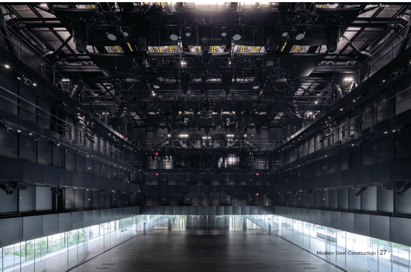
above: The side gantries can move 10½ ft toward the center of the hall, and the rear gantries can move up to 44½ ft toward the stage.
