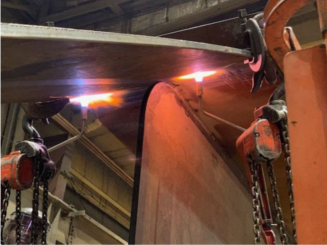
Figure C3.3.1 - Fabrication of a Rounded Top Flange Corner (High Steel LLC, 2023)
