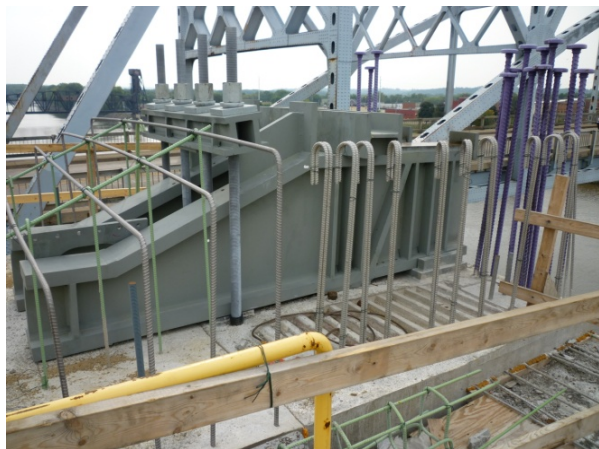
Figure 9: Support beams were inserted into the temporary knuckles after erection
