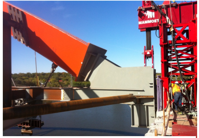
Figure 20: Lift operation is completed
