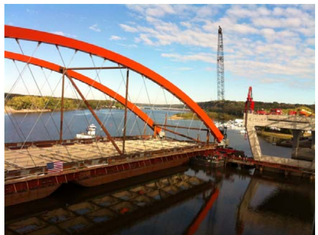
Figure 10: Temporary bracing was used during erection to stabilize the arch ribs.
