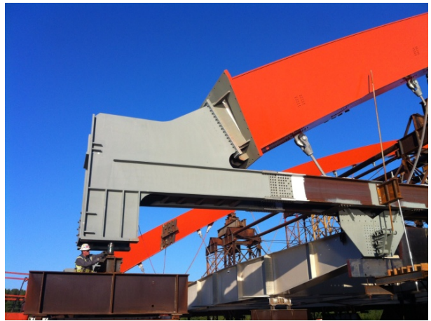
Figure 8: Temporary steel knuckle and tie.
