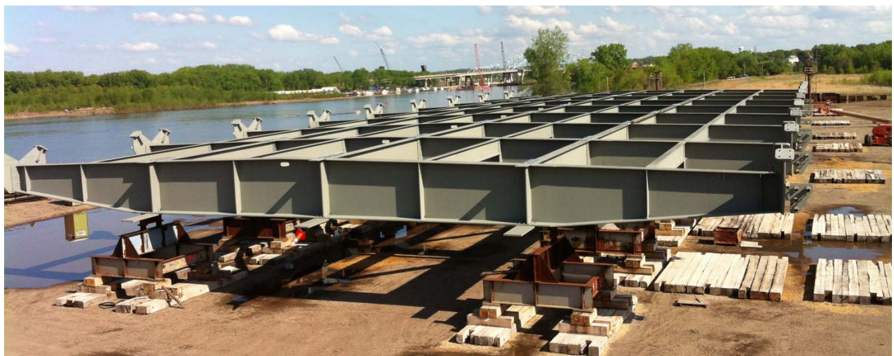
Figure 4: Independent steel grillage floor system at off-site erection yard.
