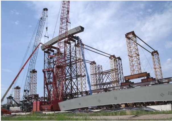
Figure 11: Center arch segment placement and fixed center tower support
