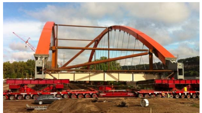
Figure 12: Arch supported by SPMT's ready for transport to barges.
