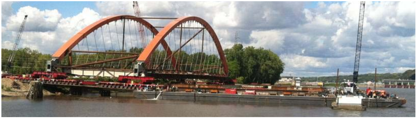
Figure 13: Arch is loaded on to ballasted barges.
