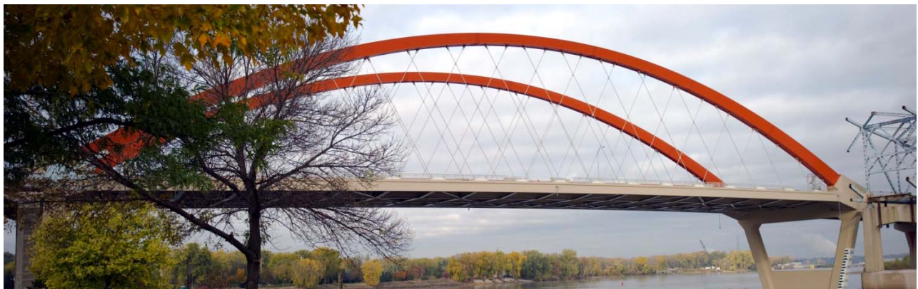
Figure 1: View of the completed free standing tied arch structure
