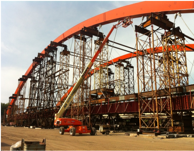
Figure 7: Off-site erection of main span.
