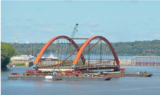
Figure 15: Barge move out to mooring area
