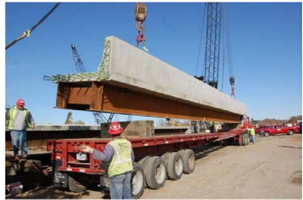
Figure 10: Typical Module Lifting
