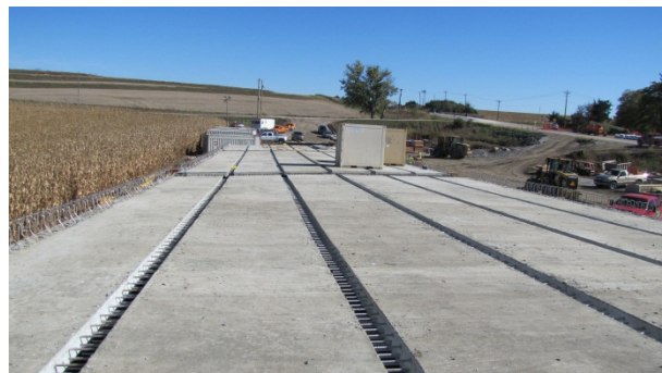
Figure 8: View of Fabricated Modules from Top of Deck
