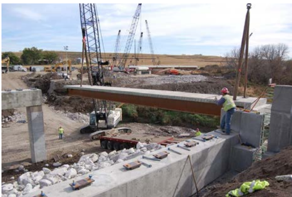
Figure 11: Module Placement at Keg Creek
