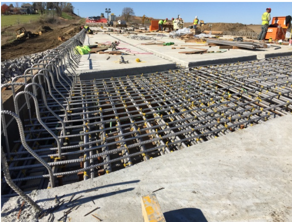
Figure 16: Transverse Deck Closure - Little Silver Creek
