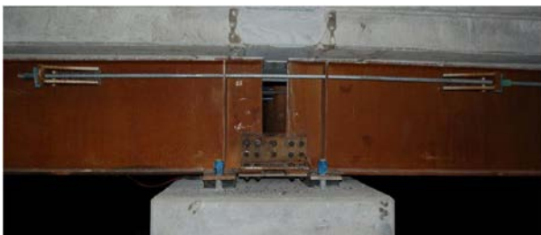
Figure 17: Bolted Tie and Post-Tensioned Detail - Keg Creek
