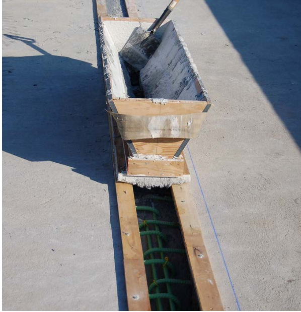
Figure 13: UHPC Longitudinal Joint - Keg Creek
