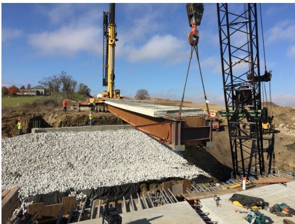
Figure 12: Module Placement at Little Silver Creek
