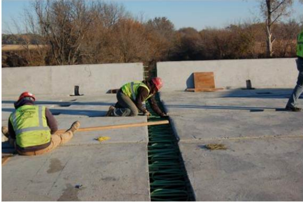
Figure 15: Transverse Deck Closure - Keg Creek
