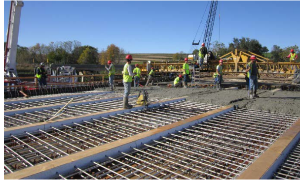
Figure 6: Module Deck Casting
