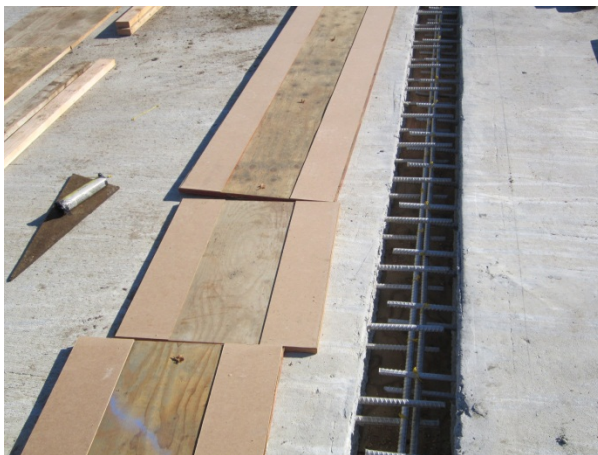
Figure 14: UHPC Longitudinal Joint - Little Silver Creek
