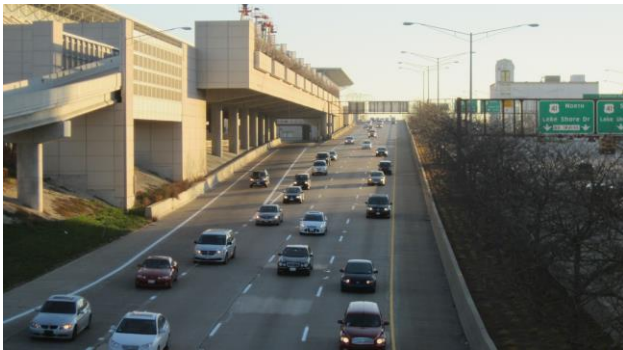
Figure 5: Existing SB I-55 next to MP West Bldg.
