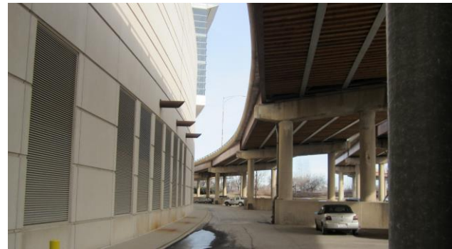
Figure 7: Existing Ramp SW by MP South Bldg.
