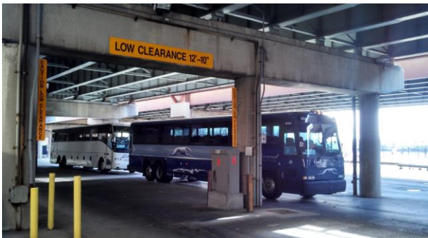
Figure 6: Existing Piers in MP Bus Staging Area
