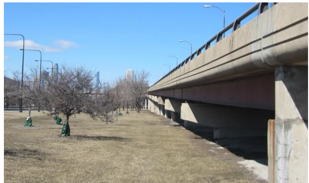
Figure 12: Existing Tangent Spans of Ramp NW
