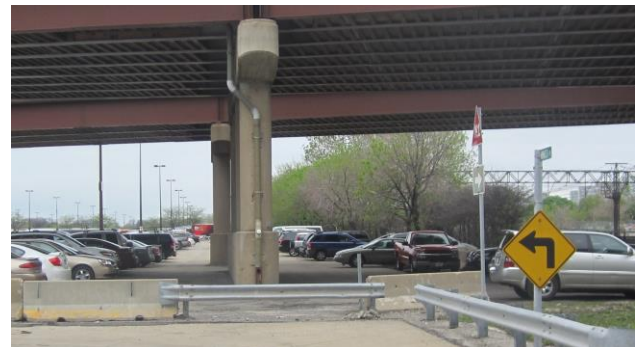
Figure 8: Existing Piers in MP Parking Lot Aisles
