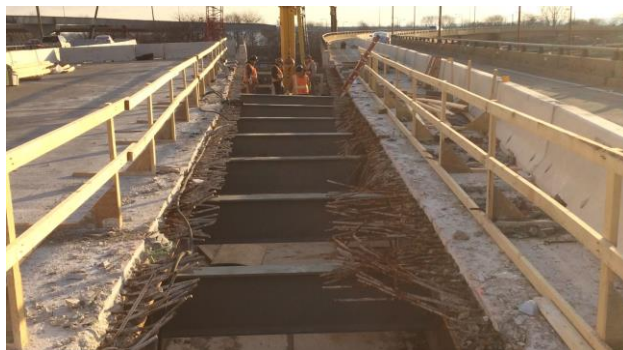
Figure 22: Gore Widening at Existing Ramp EN
