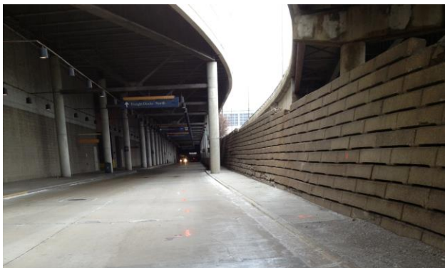
Figure 10: Existing Crib Wall east of Moe Drive
