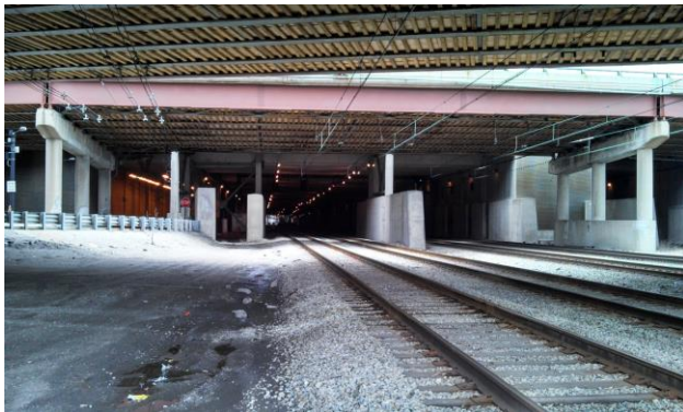
Figure 9: Metra Catenary Lines below Ramp SW
