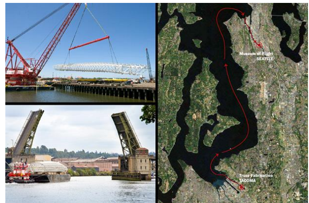
Figure 15 - The T. Evans Wyckoff Memorial Bridge in Seattle, WA, USA by Magnusson Klemencic and SRG Partnership makes a clear span across the 6 lane street in order to avoid the need for a central pier. Although the installation is over land, the route from the steel fabricator to the site required innovation in order to maximize the level of prefabrication of the curved tubular members.
