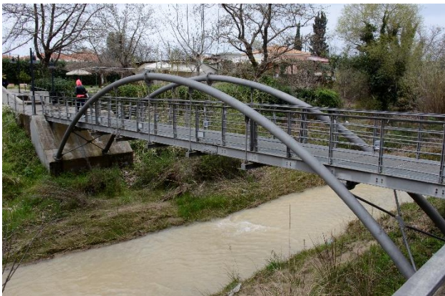
Figure 7 - This simple pedestrian bridge in Olympia, Greece is fabricated from galvanized steel. The bridge was shipped in two pieces and is joined at the center of the arch and across the deck directly below. The corrosion protection system that also serves as the architectural finish suits the more rugged situation in the archeological site. Photo by author.
