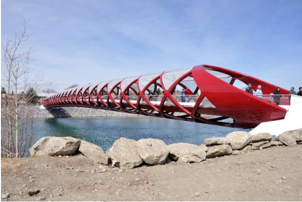
Figure 19 - The Peace Bridge in Calgary, AB, Canada designed by Santiago Calatrava uses brake forming to create the curved box sections. Photo by author.
