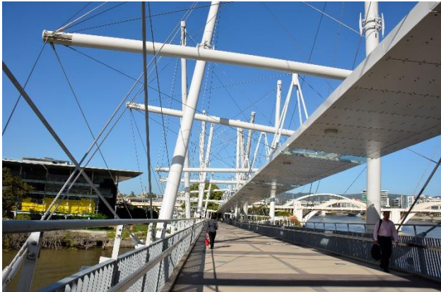
Figure 1 - The Kurilpa Bridge in Brisbane, Australia, by Cox Rayner Architects with Arup is a fine example of the exploitation of AESS to facilitate an exciting connection over the Brisbane River that separates the city. This tensegrity based structure makes a clear span across the river as no mid span supports were possible. Photo by author.
