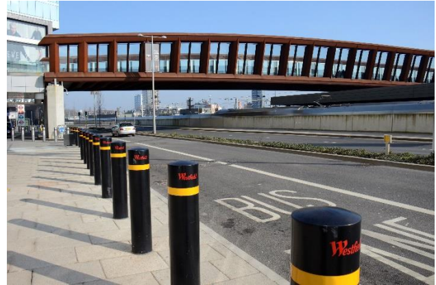
Figure 10 - Stratford Town Center Link , designed by Knight Architects with Buro Happold makes extensive use of custom bent and fabricated weathering steel plate. The bridge spans across a roadway as well as rail tracks. It is noted as the first launch of a bridge in the United Kingdom over live rail tracks.[5] Photo by author.
