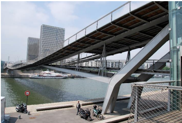
Figure 16 - The very slender profile of the Simone de Beauvoir Footbridge in Paris, France by RFR was the direct result of the requirement to transport the completed bridge to the site via barge. The clearances below the many existing bridges over the Seine required much innovation in creating a span that was extremely shallow. The bridge also had to permit adequate clearance below for the passage of vessels and was not permitted to employ an intermediate support to reduce the span. Photo by author.
