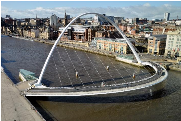
Figure 2 - The Gateshead Millennium Bridge in Newcastle, England by Wilkinson Eyre Architects accommodates pedestrians and cyclists by creating a divide down the center of the curved bridge deck. The bridge rotates to allow for the passage of boats along the river. The elements were transported to site via barges to permit the prefabrication of maximum sized elements, ease of erection and difficult access via land. Photo by author.
