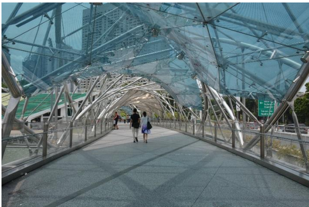
Figure 12 - The Helix Bridge in Singapore by Cox Group with Arup showcases an exquisite application of stainless steel. The selection of the material creates a very durable structure for such a moisture exposed setting. The sleek nature of the steel works well with the aesthetic of the intricate double helix structure as well as the apparent
