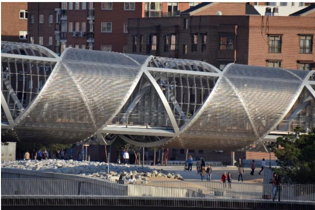
Figure 20 - The Arganzuela Footbridge in Madrid, Spain by Dominique Perrault uses un-remediated butt welds to create the corners on the custom box sections. The curved surfaces have been plate rolled. This bridge used extensive site welding to assemble the components and so the decision to leave the welds “as is” provided
