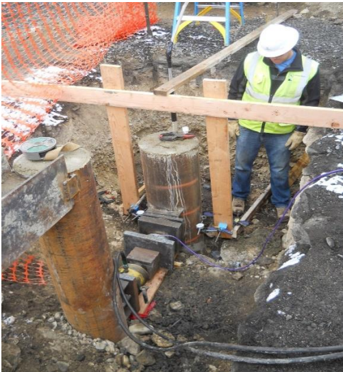
Figure 13: Pile lateral load test
