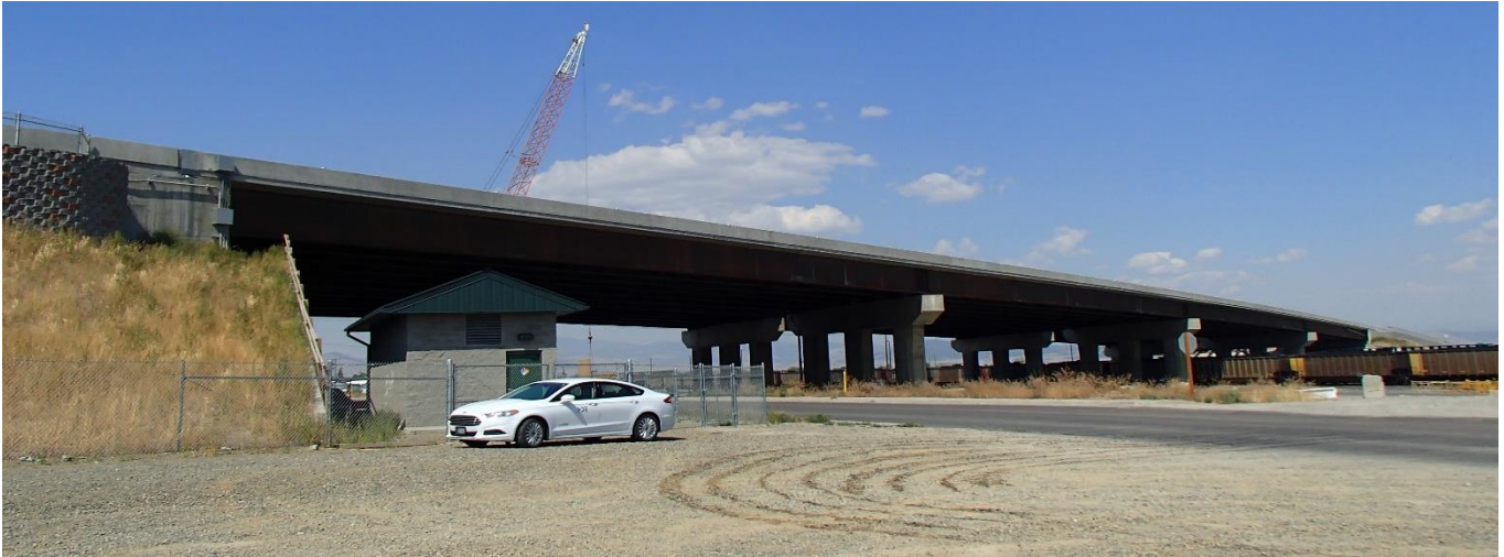
Figure 16: Completed northbound bridge
