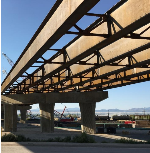
Figure 15: Northbound Bridge – Erected Girders
