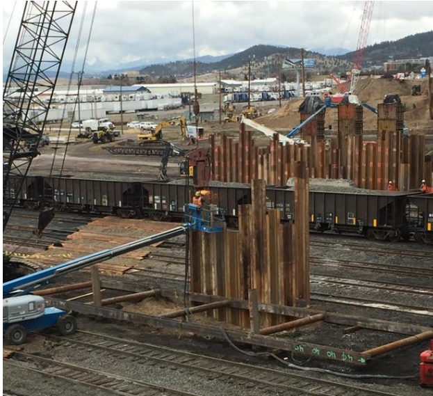
Figure 10: Bridge foundation construction
