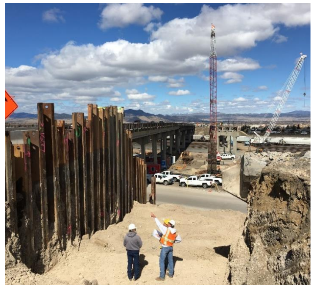
Figure 9: Temporary shoring used to support the roadway during construction.
