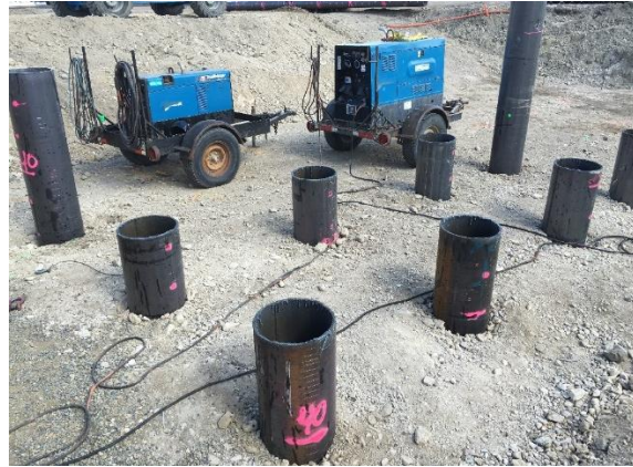
Figure 14: Installation of bridge piles during construction
