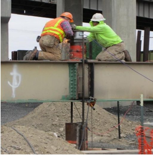
Figure 12: Pile uplift load test
