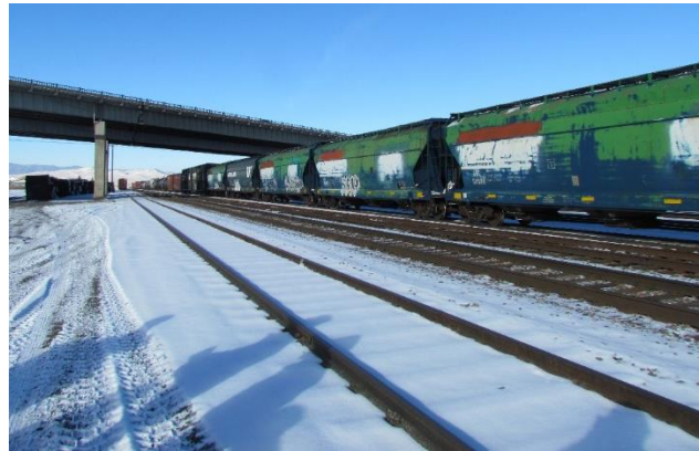
Figure 3: MRL rail yard
