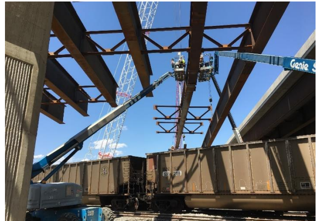
Figure 8: Erecting girders in the rail yard
