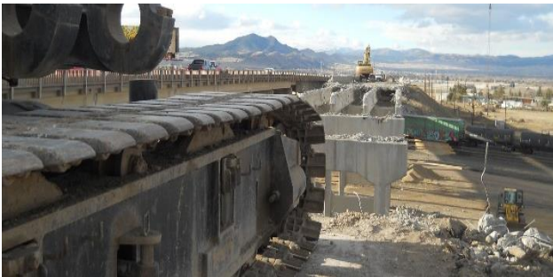
Figure 7: Existing bridge demolition
